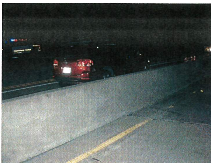
Center Divider Wall of Interstate 210 Highway
