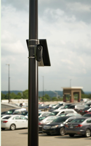
Solar & Existing Pole
