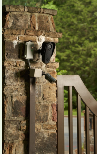
Electric & Existing Structure / Pole
