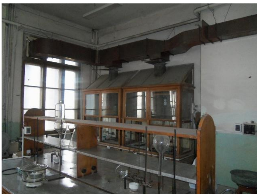
Figure 11-5 Chemical hoods in Chemistry Lab. Reported to be functioning.
