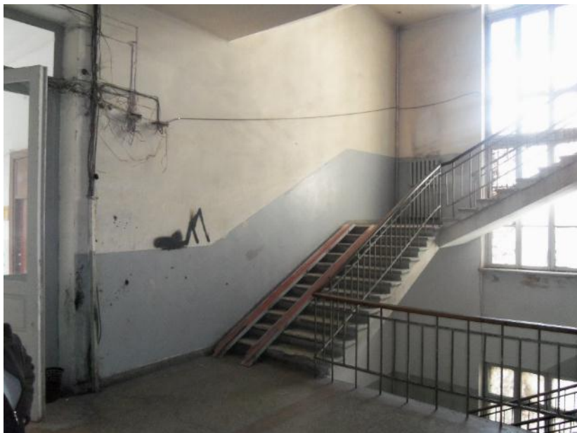
Figure 11-4: Foyer stairwell in Chachavadze building. Note the electrical cabling is messy. The stairs have wheelchair ramps.
