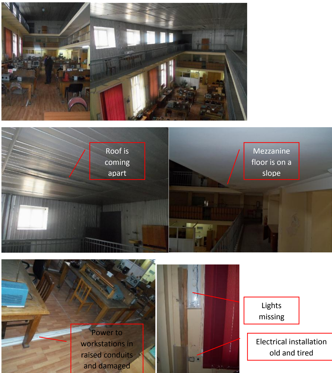
Figure 11-3: Example space of Approximately 150 m 2 with 2 tier mezzanine floor at Chachavadze building, currently used as physics laboratory. The roof has some damage and the top tier of the overhung mezzanine has a distinct lean and what appears to be water damage raising structural concerns. Lights are missing and electrical wiring is old. Windows are also old two pane style.
