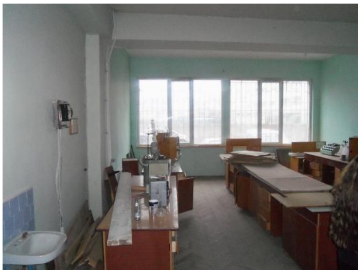
Figure 12-2: Space requiring refurbishment, note exposed electrical installation on left, all services to this space are tired and likely require refurbishment.
