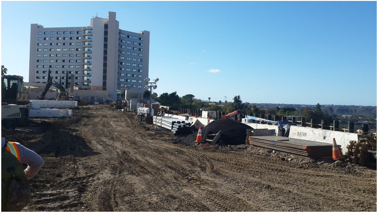
Last field visit, SDSU New Student Resident Hall – Clark Construction (Photo by: Dr. Shishinashvili)
