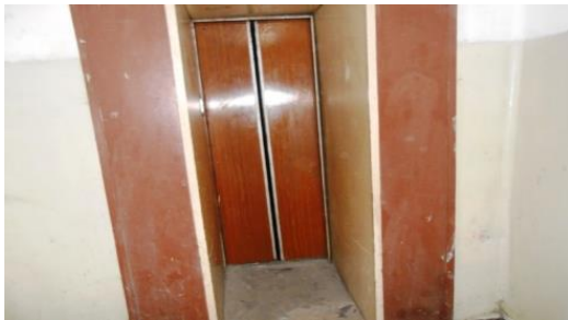
Very Narrow Elevator
