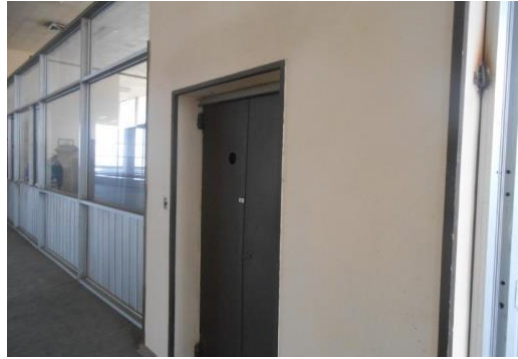
The elevator is abolished on 6th floor
