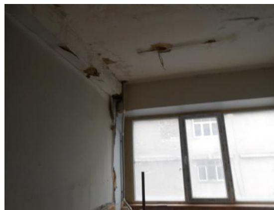
Leakage behind the ceiling
