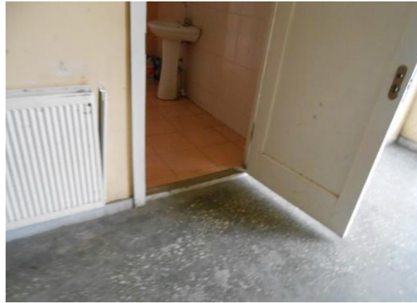
Obstructions for disabled people to get the washroom
