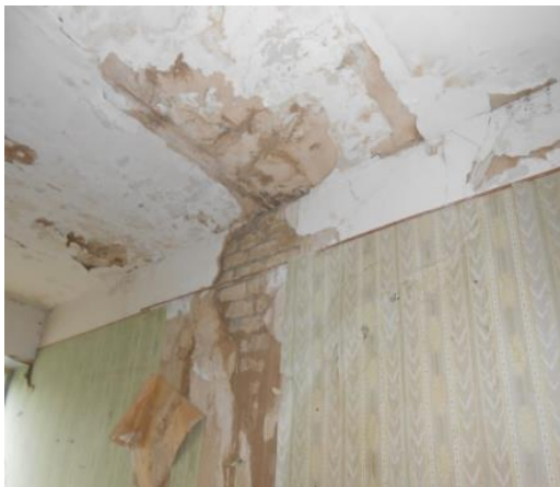
Leakage on the wall and ceiling is occurred
