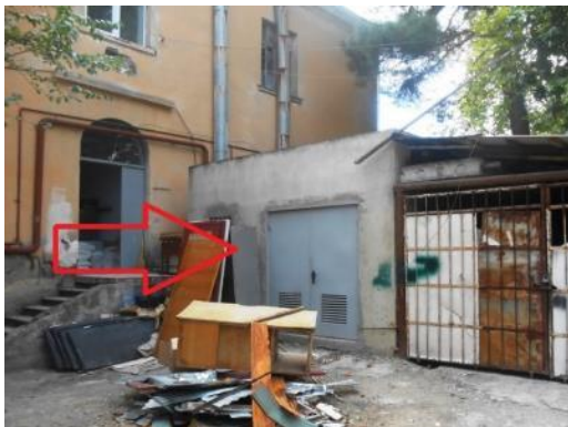
Gas boiler should be relocated
