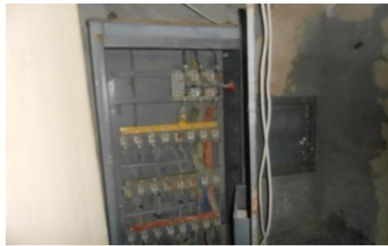
Electric Power Distribution Box
