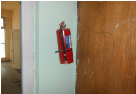
Fire extinguisher is available (expired)
