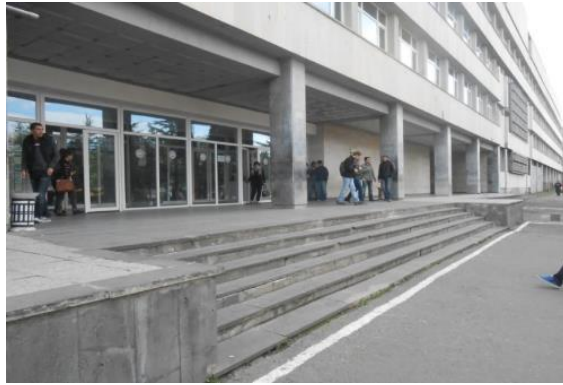
Entrance, NO accessibility for disabled people
