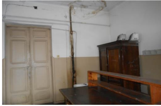
Corroded steel pipes in laboratory
