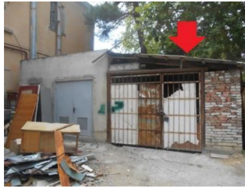
Asbestos roofing of the storage
