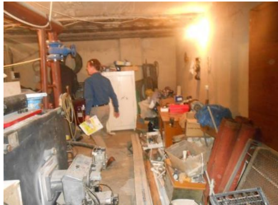
Gas boiler should be relocated
