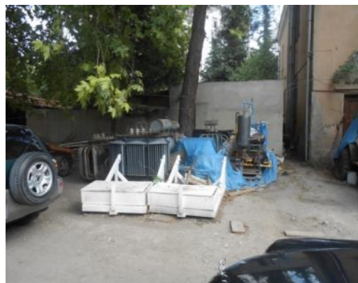
Generator is just put in the yard
