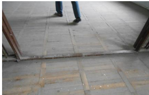
Obstruction for disabled people
