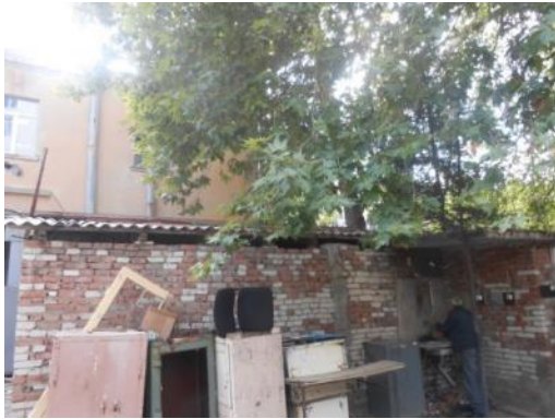
Asbestos roofing of the storage
