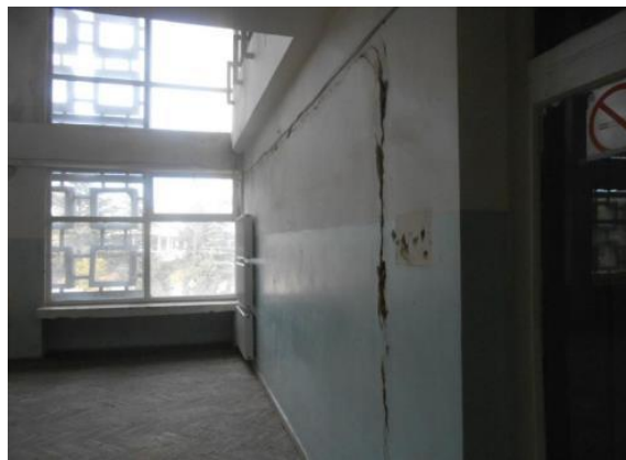
Cracks on the walls
