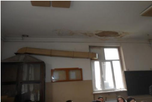
Ventilation arranged in laboratory
