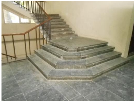
Inside Stairs, NO accessibility for disabled people
