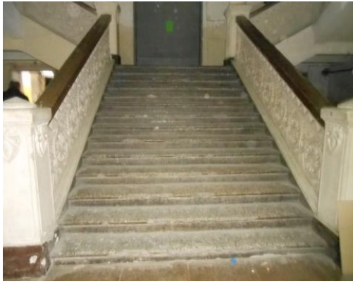
Inside main Stairs, NO accessibility for disabled people
