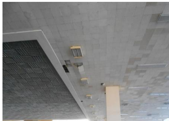
Ceiling tiles arrangement
