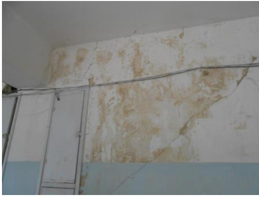
Mold and Moisture on the wall
