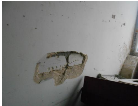
Brick Partition Wall between the laboratories
