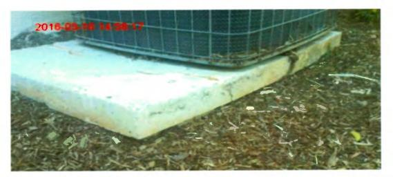
Often inspectors record a defect for erosion because the area under a tree or path that residence use does not have grass growing on it. This is not correct. Erosion shall be evaluated only if there is evidence of displaced soil.
