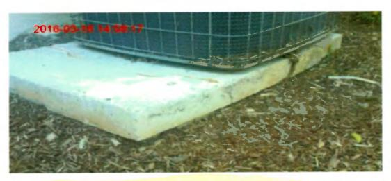
Often inspectors record a defect for erosion because the area under a tree or path that residence use does not have grass growing on it. This is not correct. Erosion shall be evaluated only if there is evidence of displaced soil.
