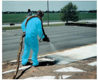
FAST Adhesive is spray-applied to the existing substrate, then insulation boards are set into the adhesive after it develops string/body.
