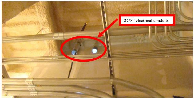
Image 3: The image above is taken inside a 3<sup>rd</sup> floor utility room beneath the rooftop mechanical area. The two electrical conduits shown in this image are stubbed down from the roof. Image 4 below shows two additional conduits on the other side of this 3<sup>rd</sup> floor utility room that run continuously to the 2<sup>nd</sup> floor electrical room.
