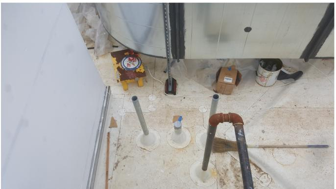
Figure 12: Eastern roof top 3" conduit rooftop penetration.
