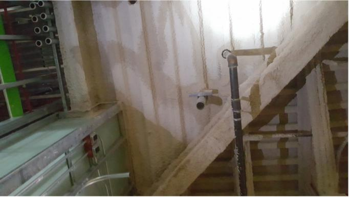
Figure 15: Eastern 3" conduit rooftop penetration inside. Note, this conduit has been extended and routed down the main electrical room.
