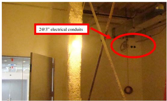
Image 4: The image above is taken inside a 3<sup>rd</sup> floor utility room beneath the rooftop mechanical area. The two electrical conduits shown in this image are stubbed out of the wall and run continuously from here to the 2<sup>nd</sup> floor electrical room.
