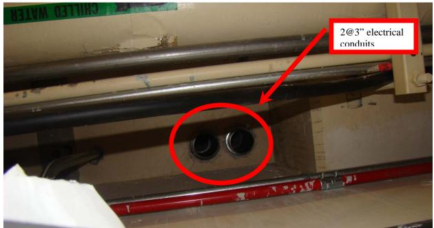
Image 1: The image above is taken inside the second floor electrical room. It shows the two empty 3" conduits penetrating through the ceiling of the electrical room.
