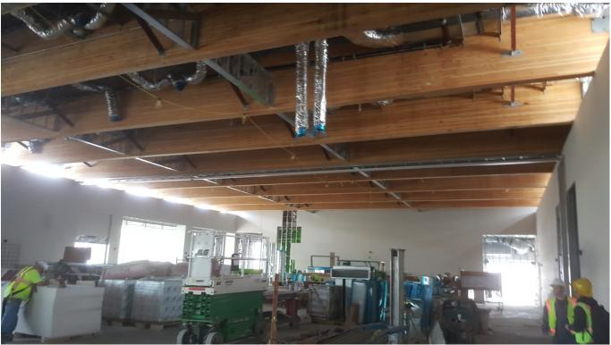
Figure 16: Gluelam beams exposed beneath upper roof area.
