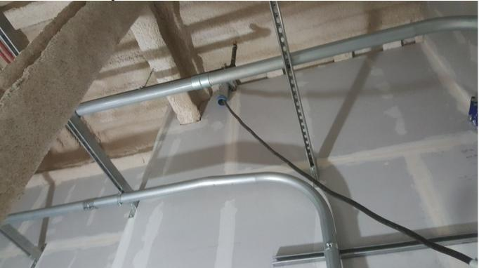
Figure 14: Western 3" conduit rooftop penetration inside. Note, this conduit has been extended and routed down the main electrical room.
