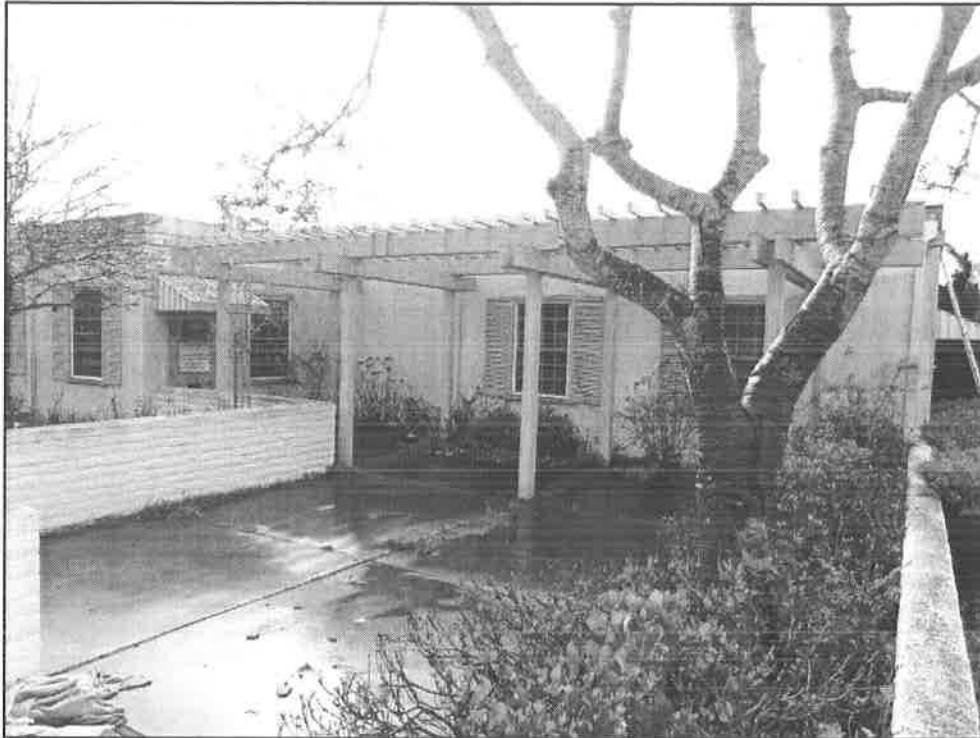
Front of building
