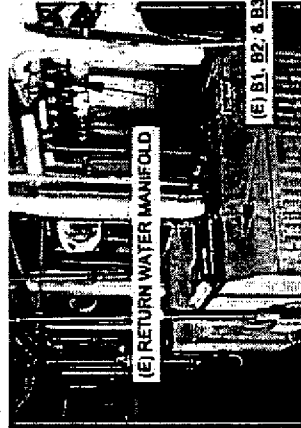
6 - SPACE HEATING BOILERS
