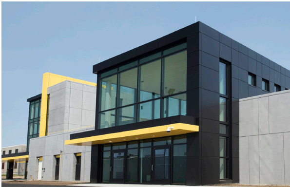
WCSO Combined Intake and Medical Unit is a high performance, climate resilient building that conforms to the MA Stretch Code.
