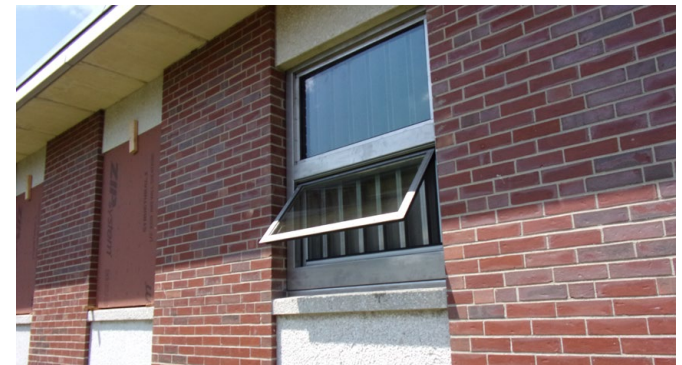
New Mock-up Window Installation
