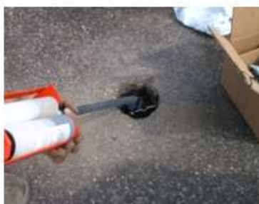
Step 3: Sensor is covered by resin
