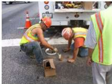
Step 3: Sensor is covered by resin
