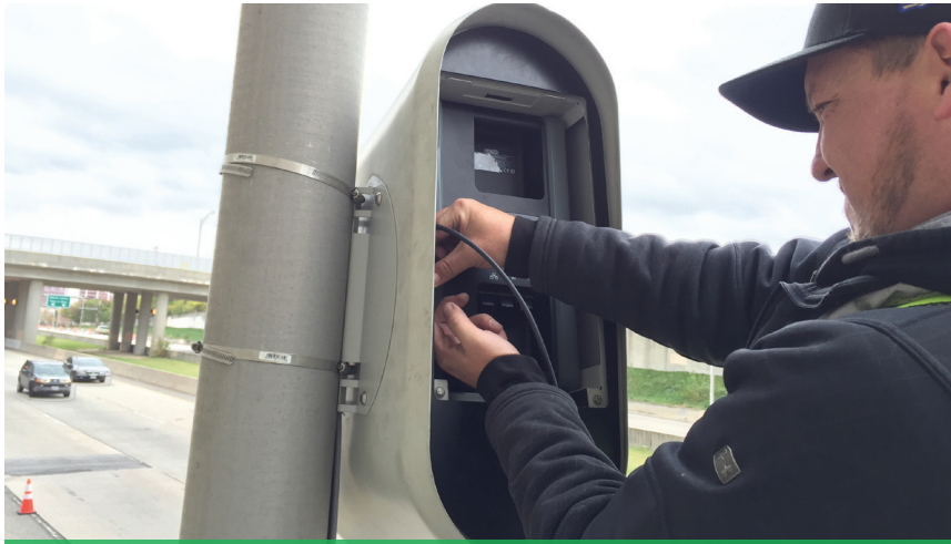
SENSYS GATSO ENGINEER PERFORMING AN INSTALL
