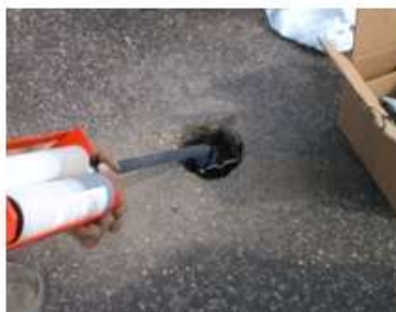
Step 3: Sensor is covered by resin
