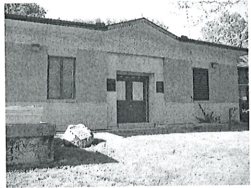
120 Springhouse Water Plant
