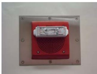
Fire alarm horn and strobe light
