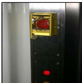
Emergency override button
