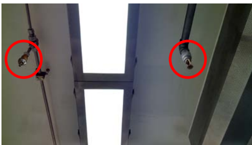
BSL-4 fire suppression system: Mist system on left and pre-action sprinkler on right
