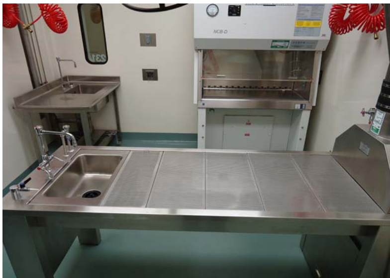
Animal necropsy room with downdraft table and Class II, B1 BSC
