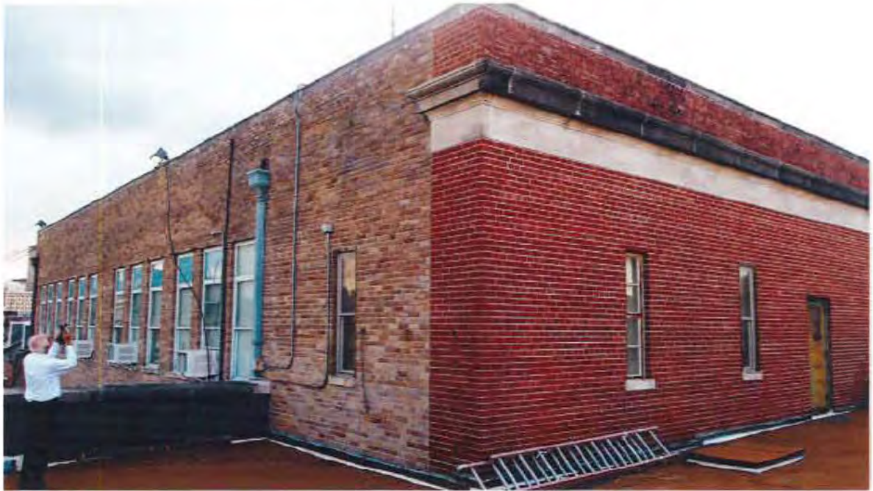
33. School, Eastern & southern elevation, looking northwest
