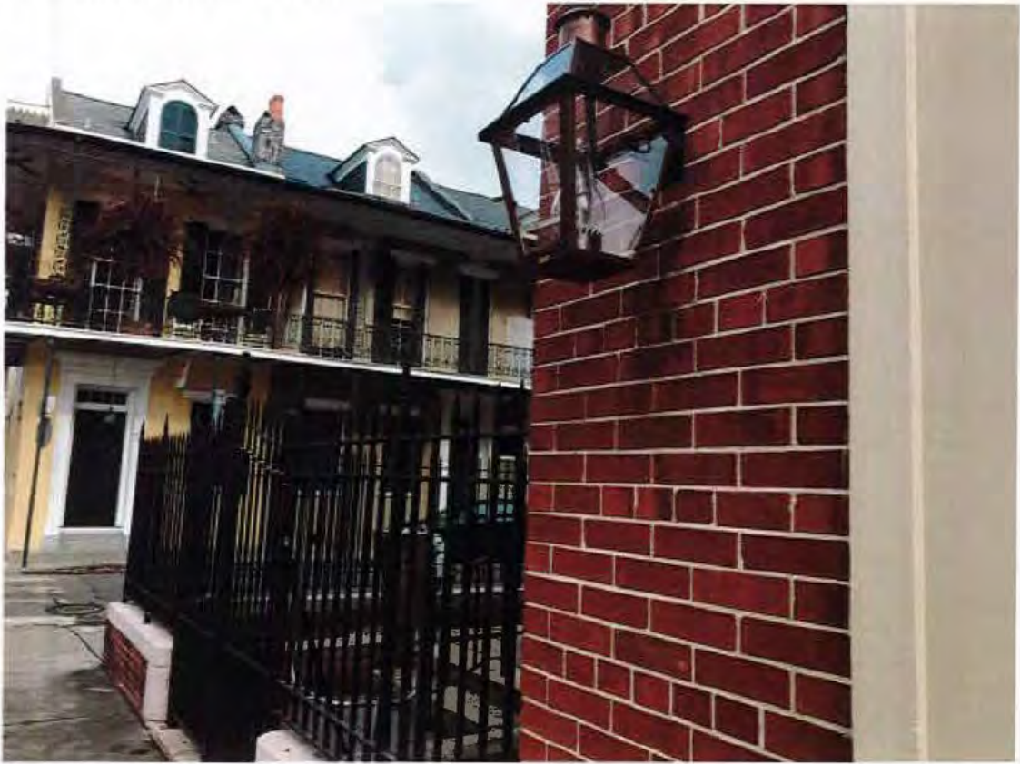
9. Convent, gate detail, looking southeast
