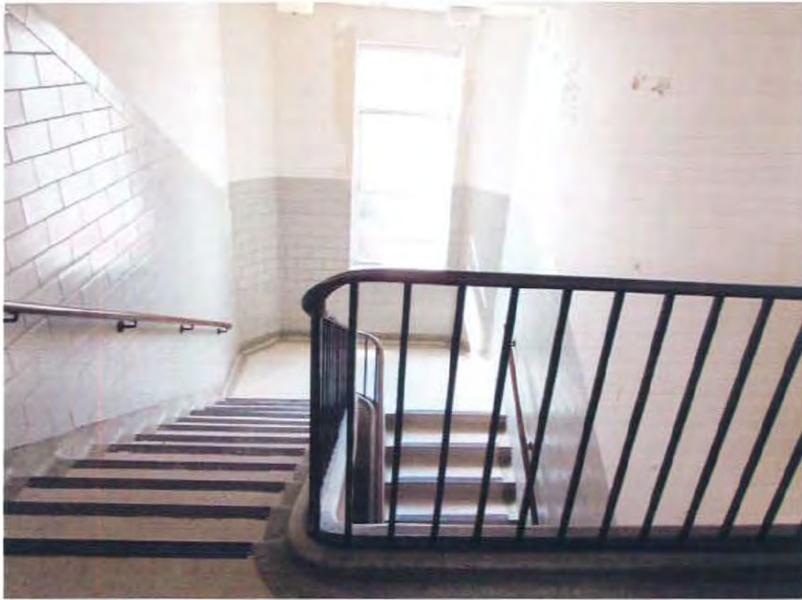
59. School. 3rd floor stair, looking north
