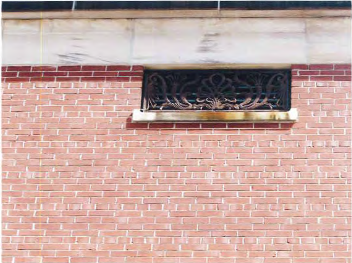
27. School, iron grille details, looking south
