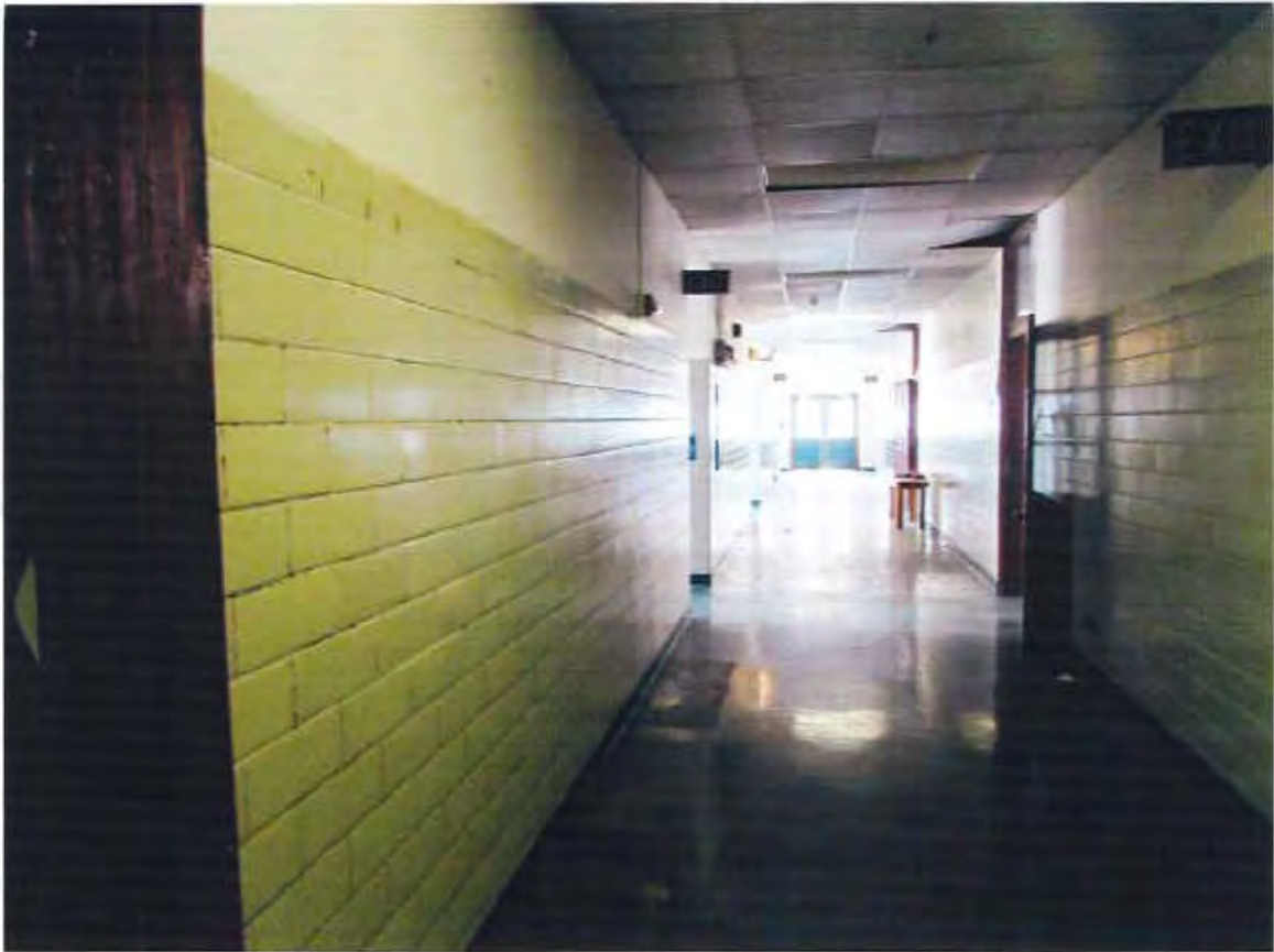
35. School, 1st floor corridor, looking west toward entry from side parking lot
