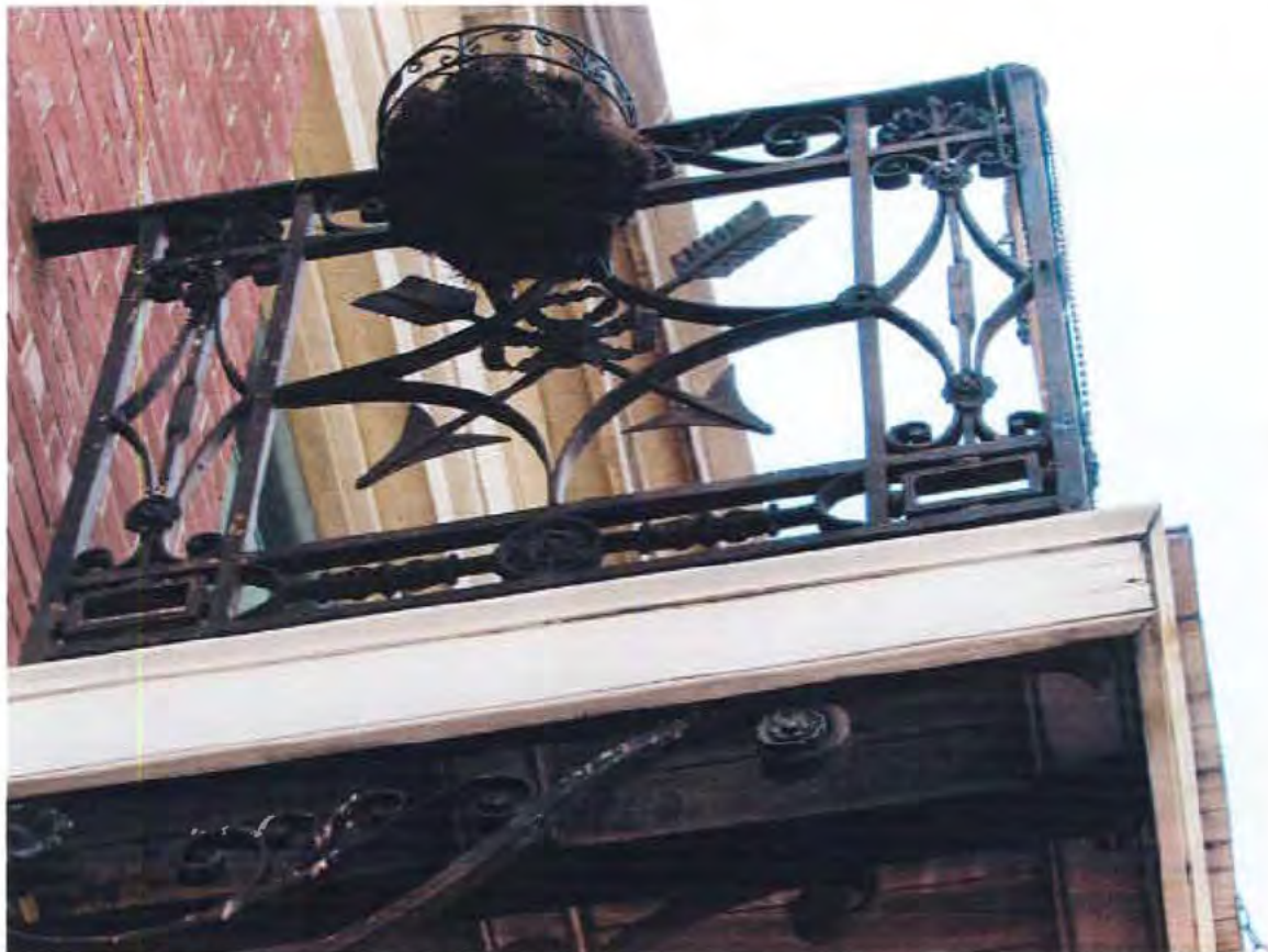
16. Convent. Balcony detail, looking north
