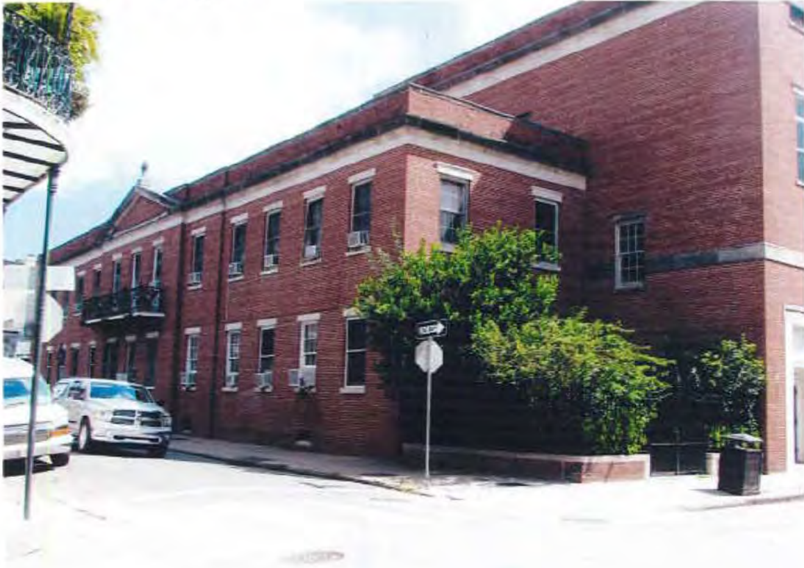
9. Convent, corner of Dauphine and Dumaine Streets, looking south
