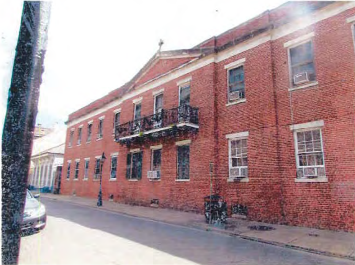
2. Dumaine Street Facade, looking southwest
