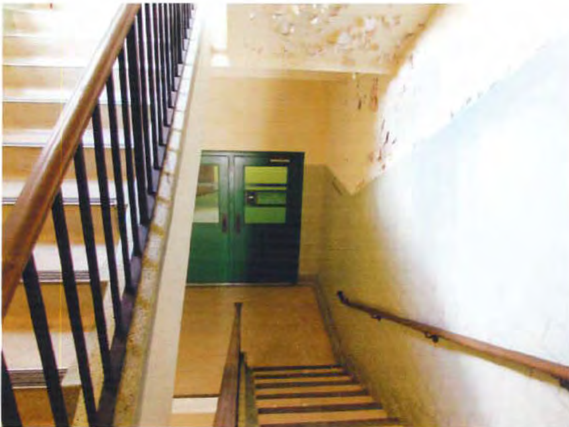
40. School, 2nd floor stair, looking north
