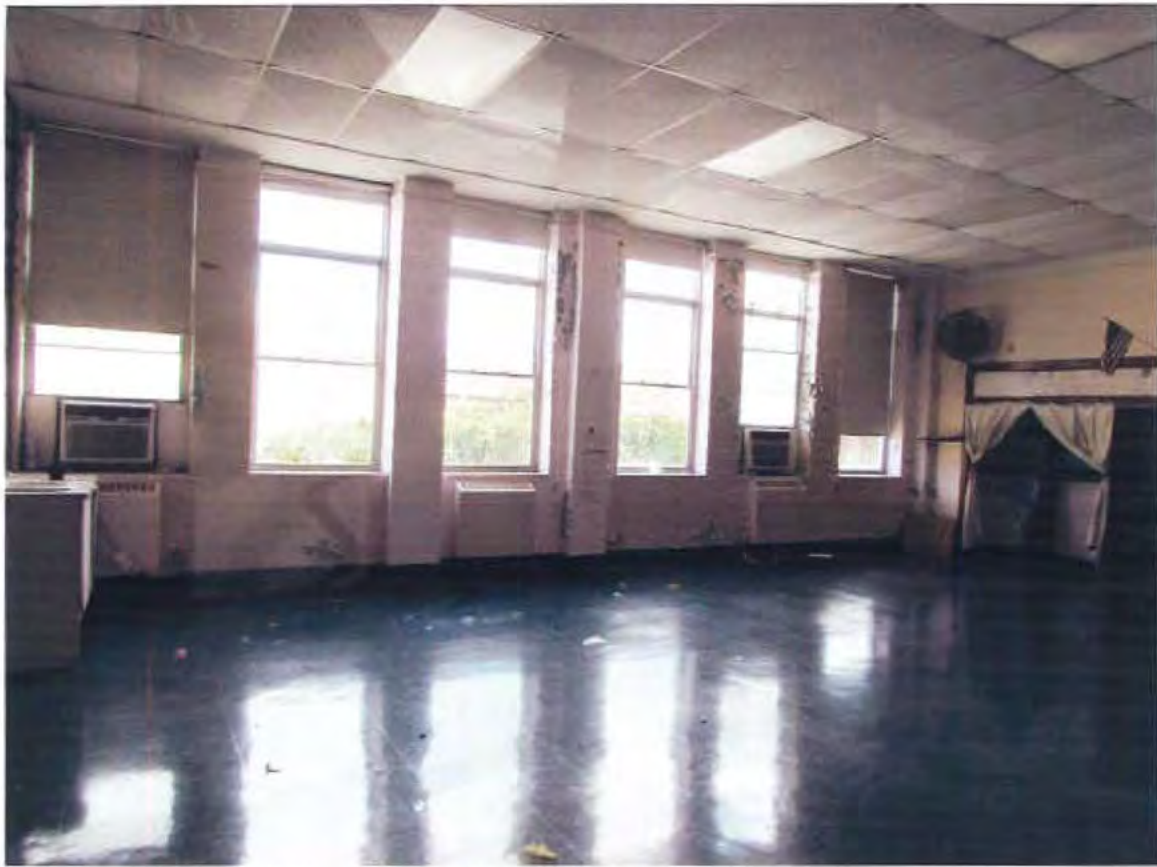
57. School 2nd floor kindergarten, looking southwest
