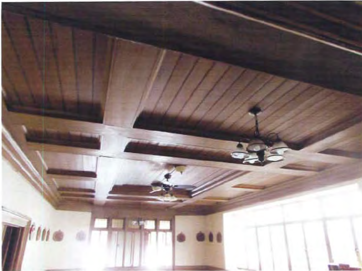
77. Chapel wood ceiling detail
