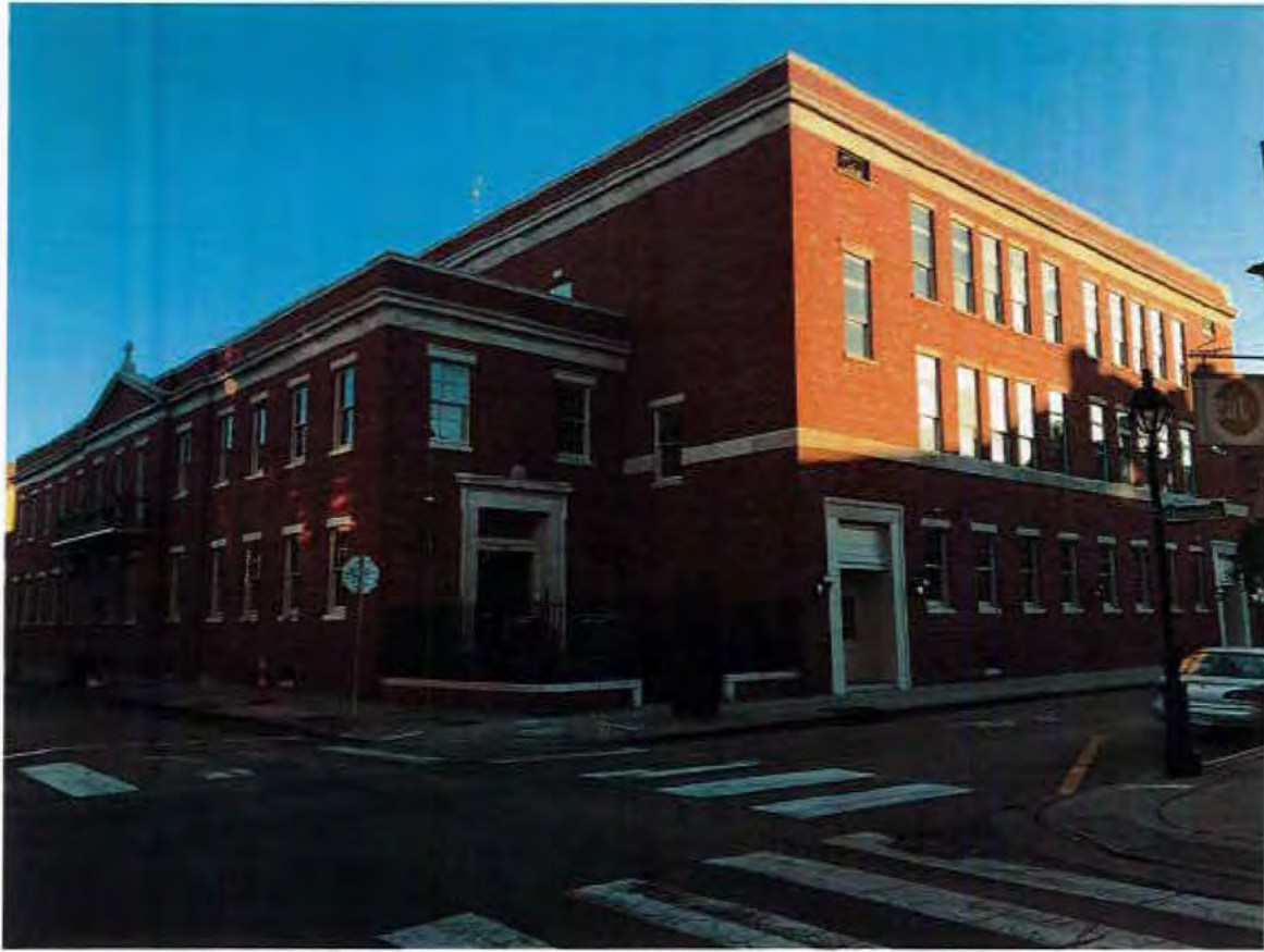
1. Dauphine & Dumaine Street Façades, looking southwest
