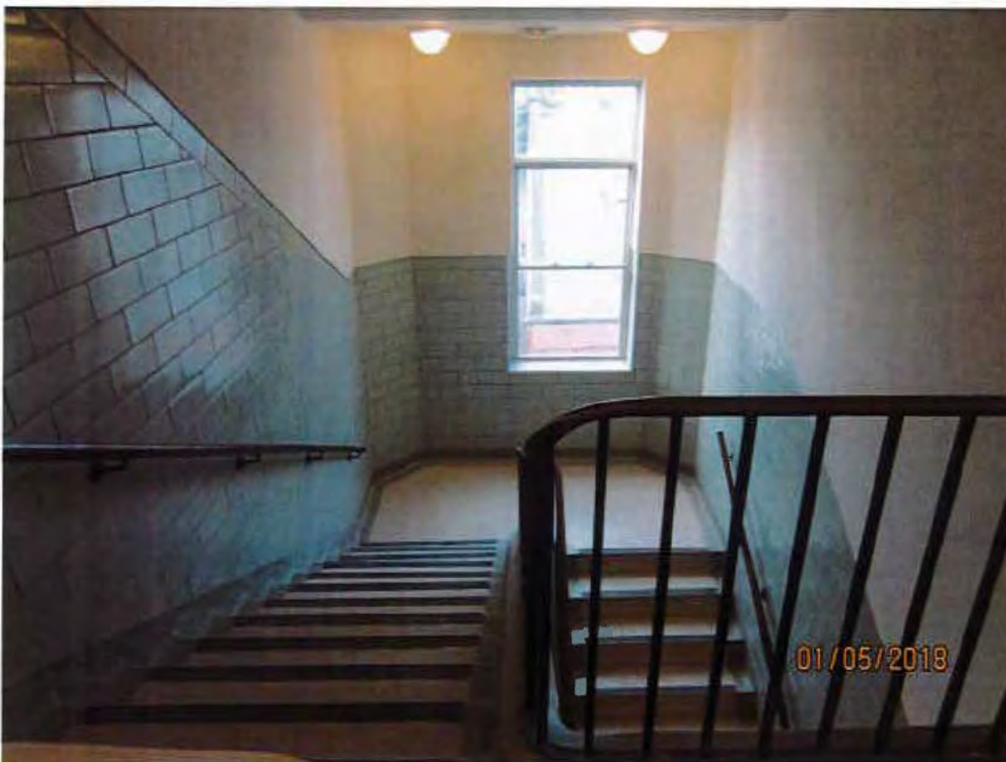
51. School, 3 rd floor stair, looking north
