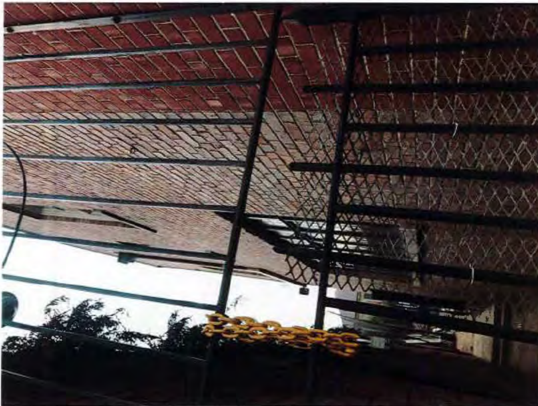
15. Convent, southern side elevation, looking west
