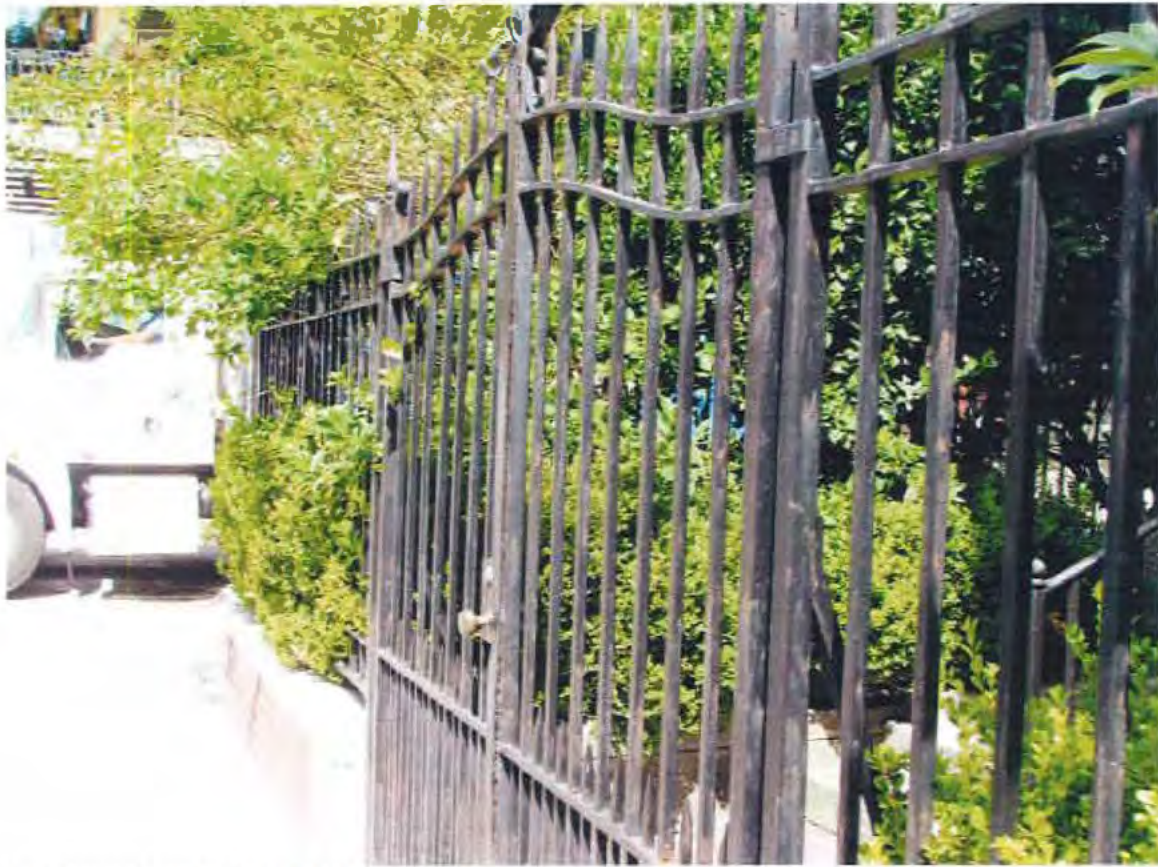
13. Convent, gate detail, looking southeast
