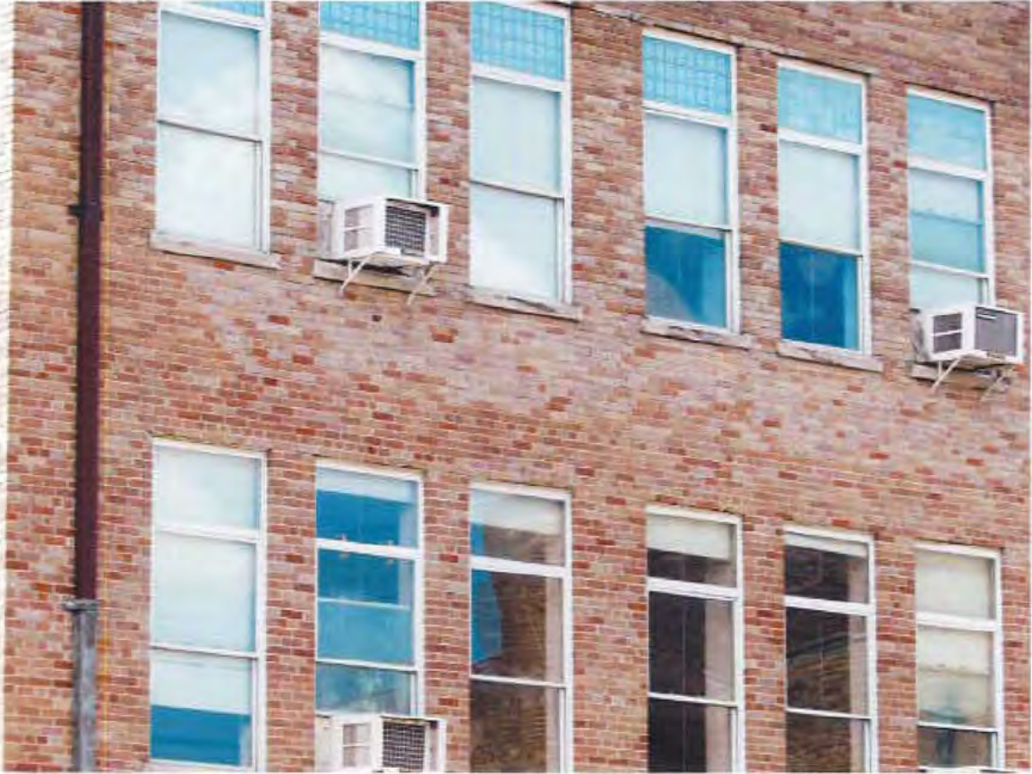
32. School, rear windows detail, looking north
