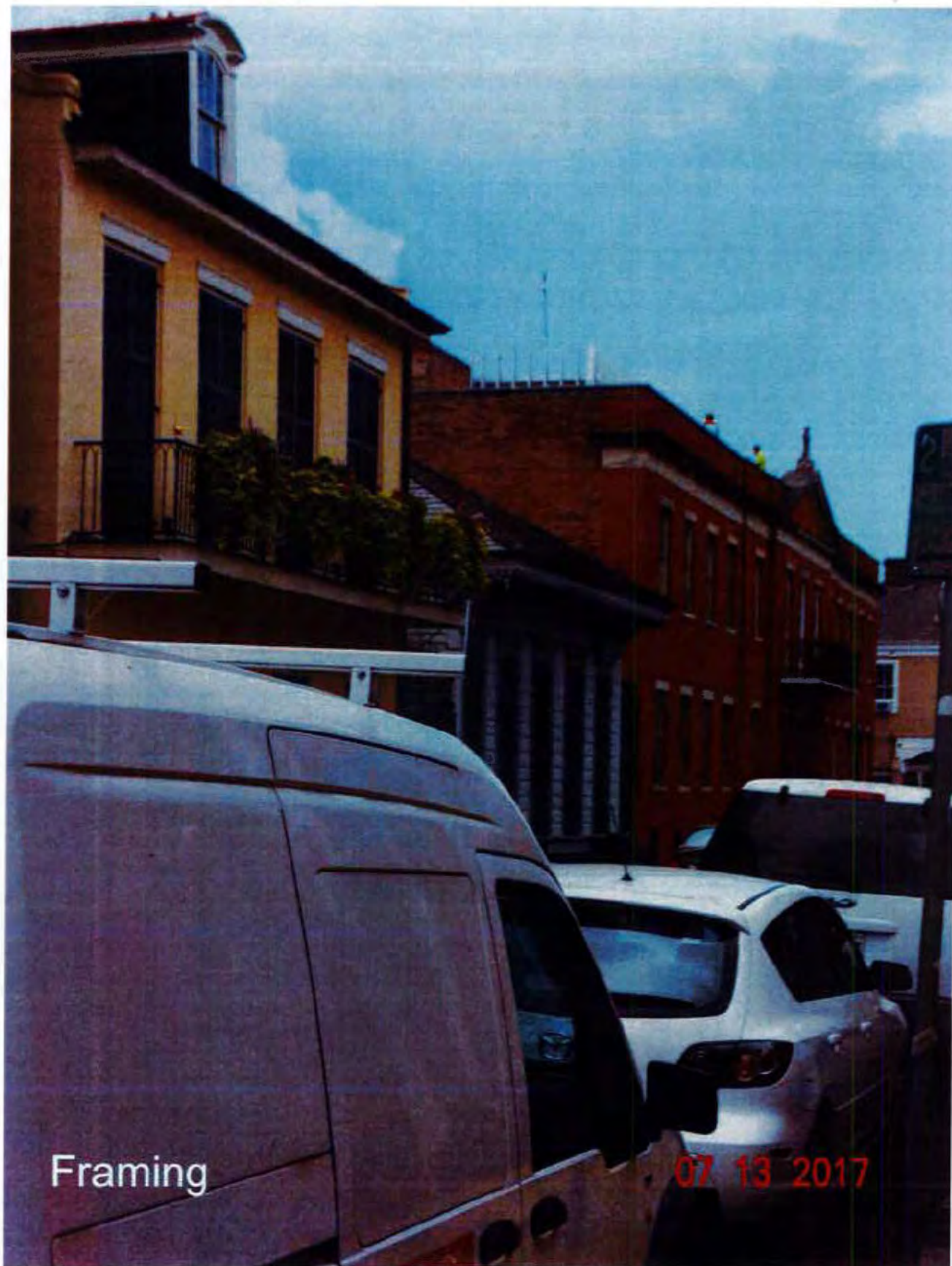
Figure 6: Construction photo of rooftop addition from the east on Dumaine Street.
