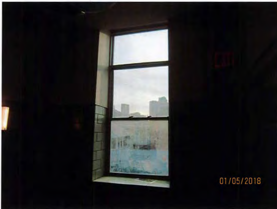
44. School, 2 nd floor corridor, western elevation window
