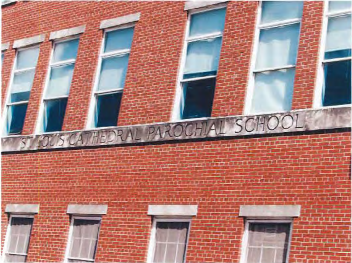
28. School. Facade detail—signage & windows
