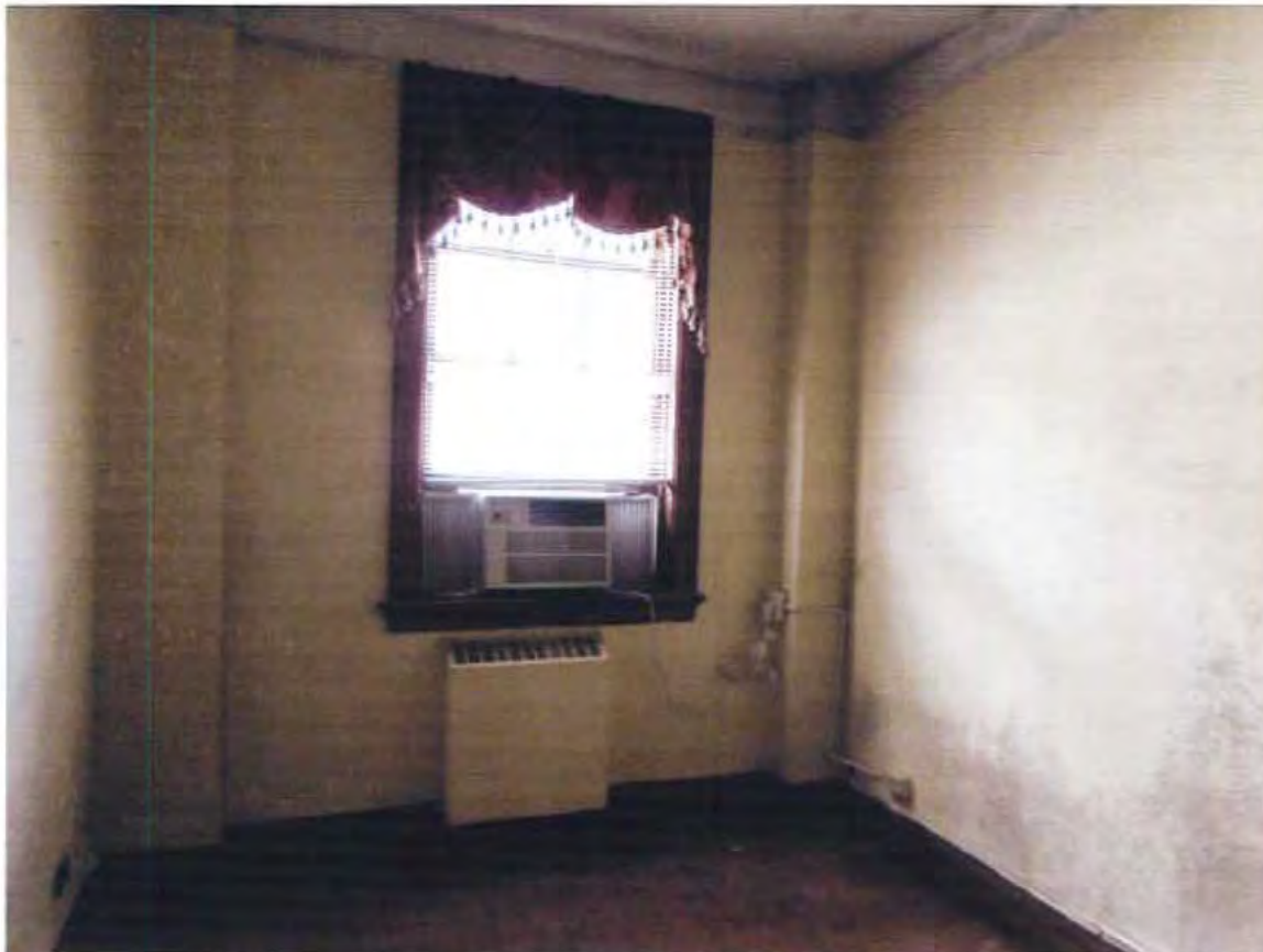
84. Convent, 1st floor, office, looking east
