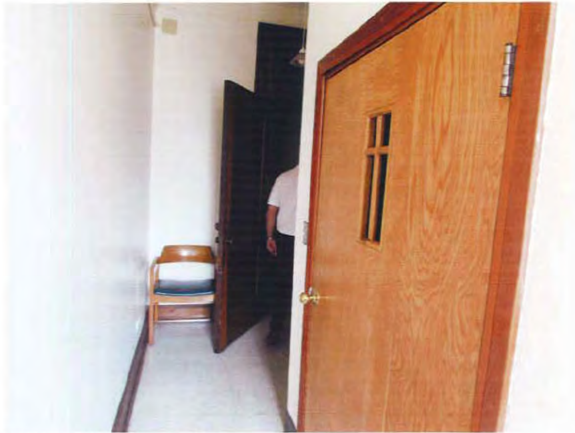
85. Convent. 1st floor elevator door
