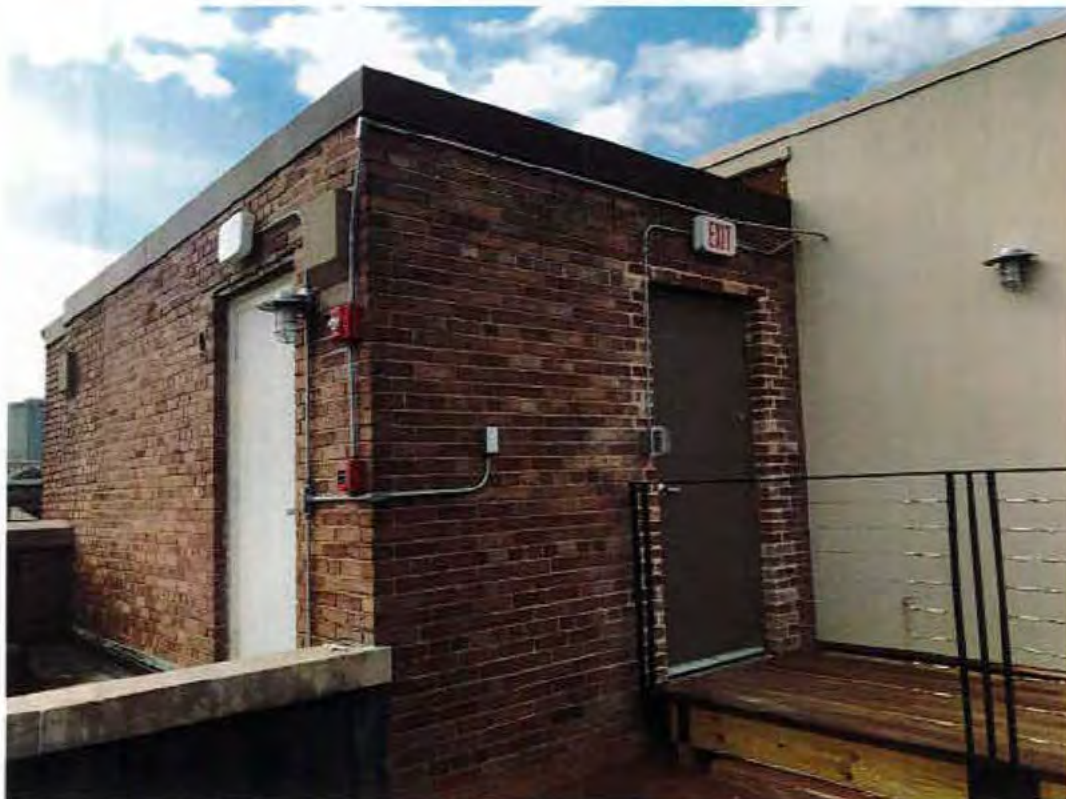
86. Convent roof, looking northwest, stair penthouse & terrace
