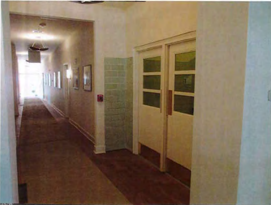
39. School, 1 st floor, looking northwest toward stair 1 & Dauphine Street entry
