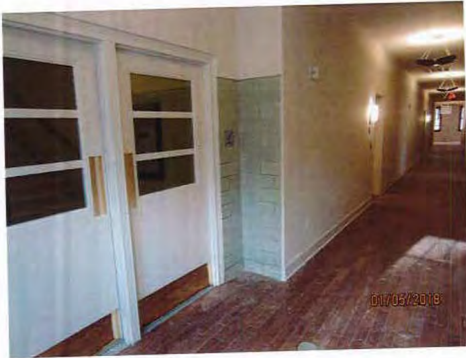
33. School 1 st floor, stair 2, looking northeast
