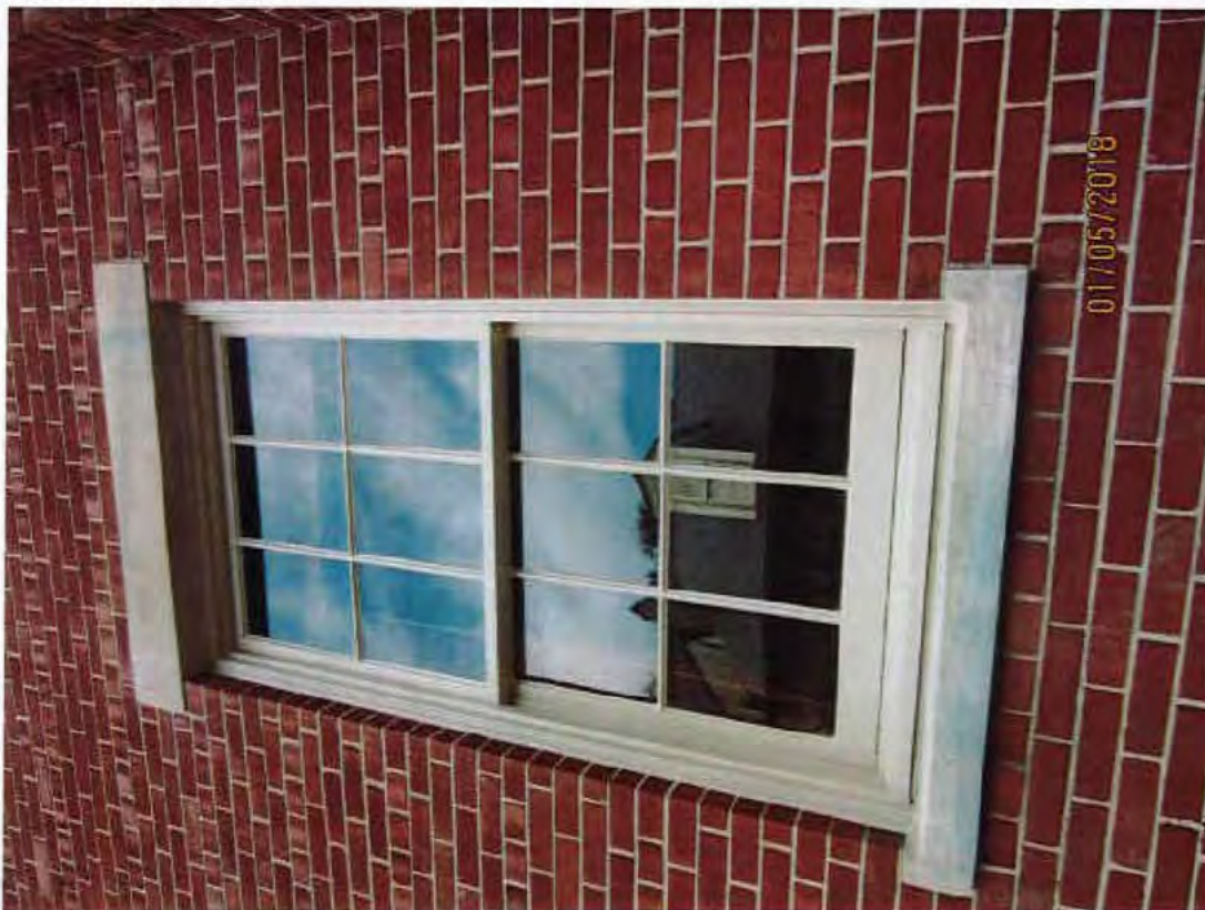
14. Convent, window detail, looking west
