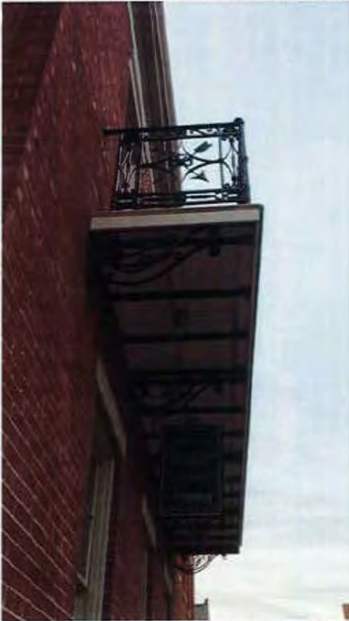
11. Convent, Balcony detail, looking north
