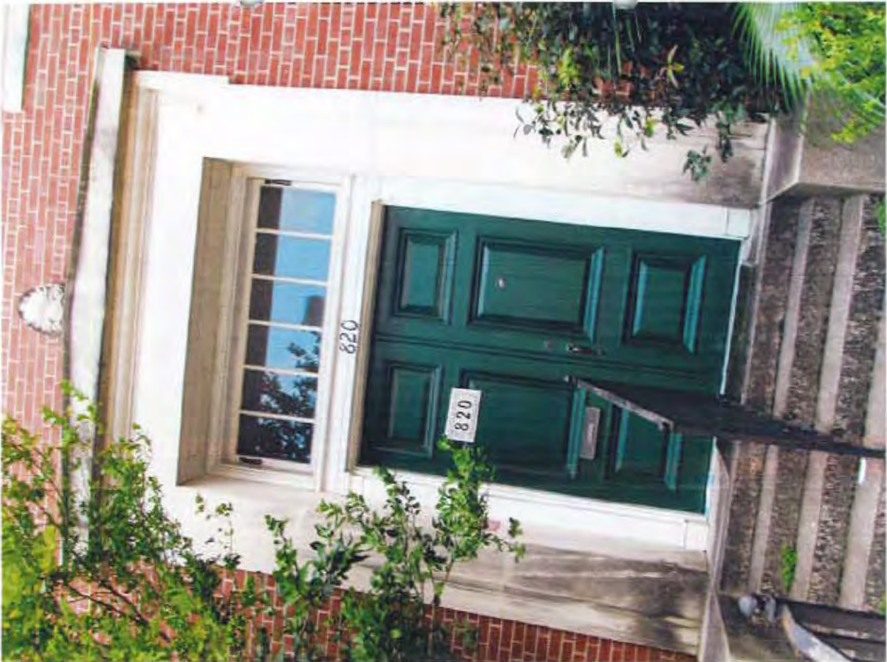
11. Convent, entry details, looking south
