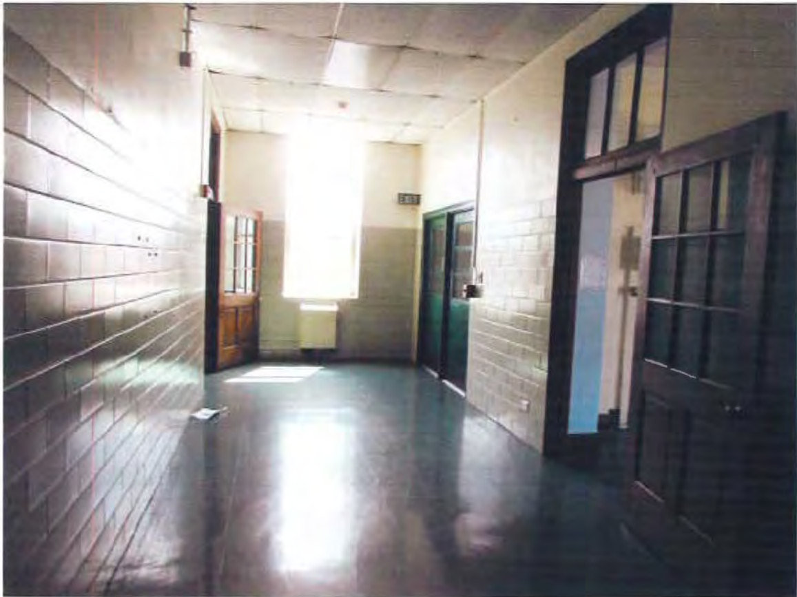
60. School 3rd floor corridor, looking west
