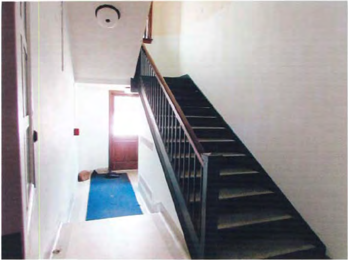
87. Convent, 1st floor, stair, looking west
