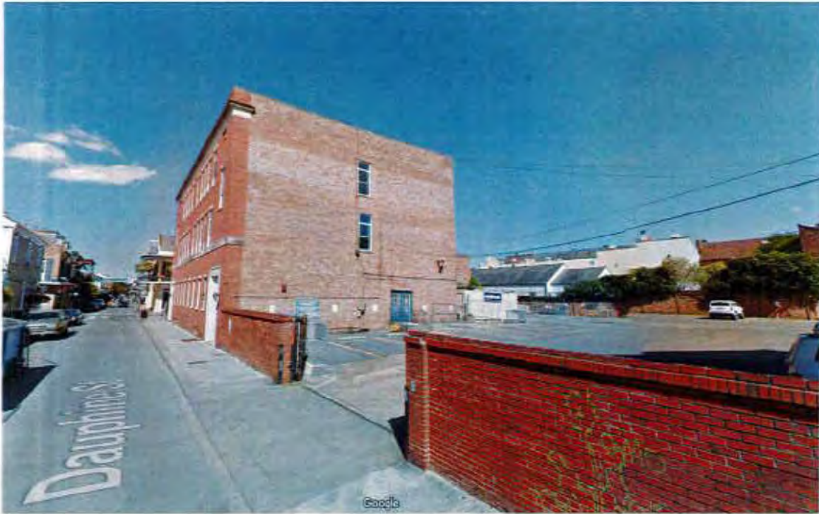
Figure 3: The Cathedral Academy from the southeast on Dauphine St., showing the parking lot where infill construction is approved.
