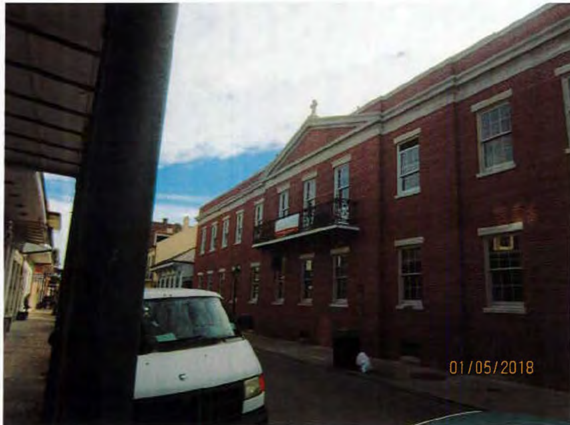
2. Dumaine Street façade, looking southwest
