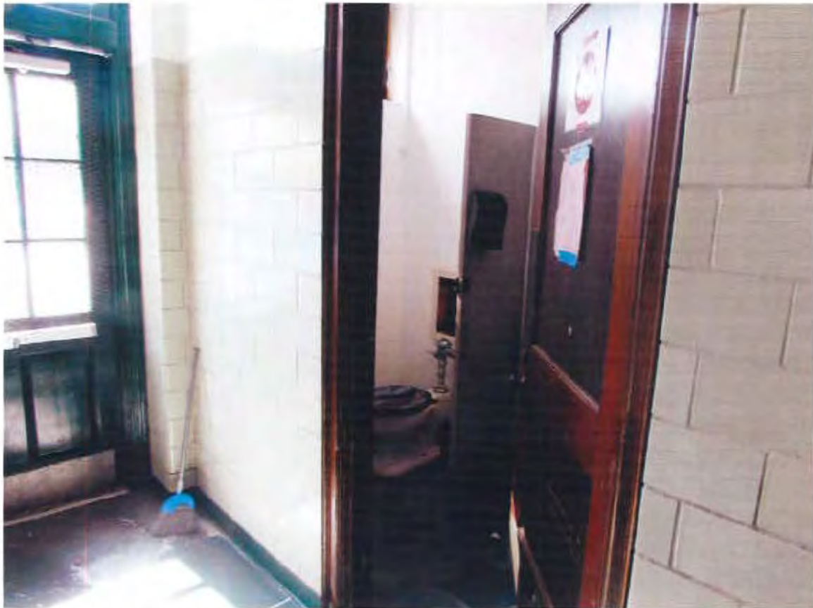
50. School, 1st floor, 3rd toilet, looking southwest
