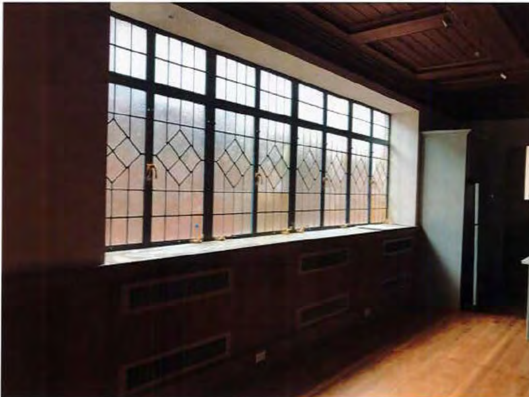
70. Chapel. Steel and glass cathedral window, looking south
