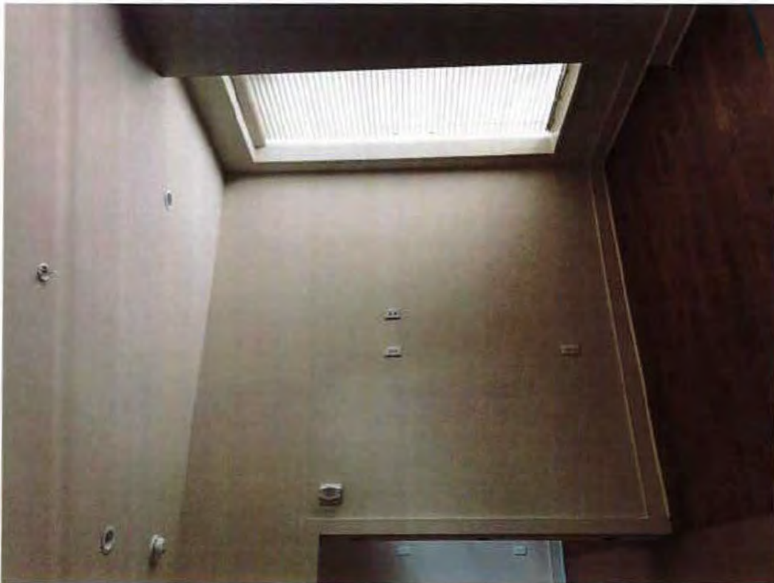
40. School, 1 st floor, boys' toilet, looking southeast, looking northeast
