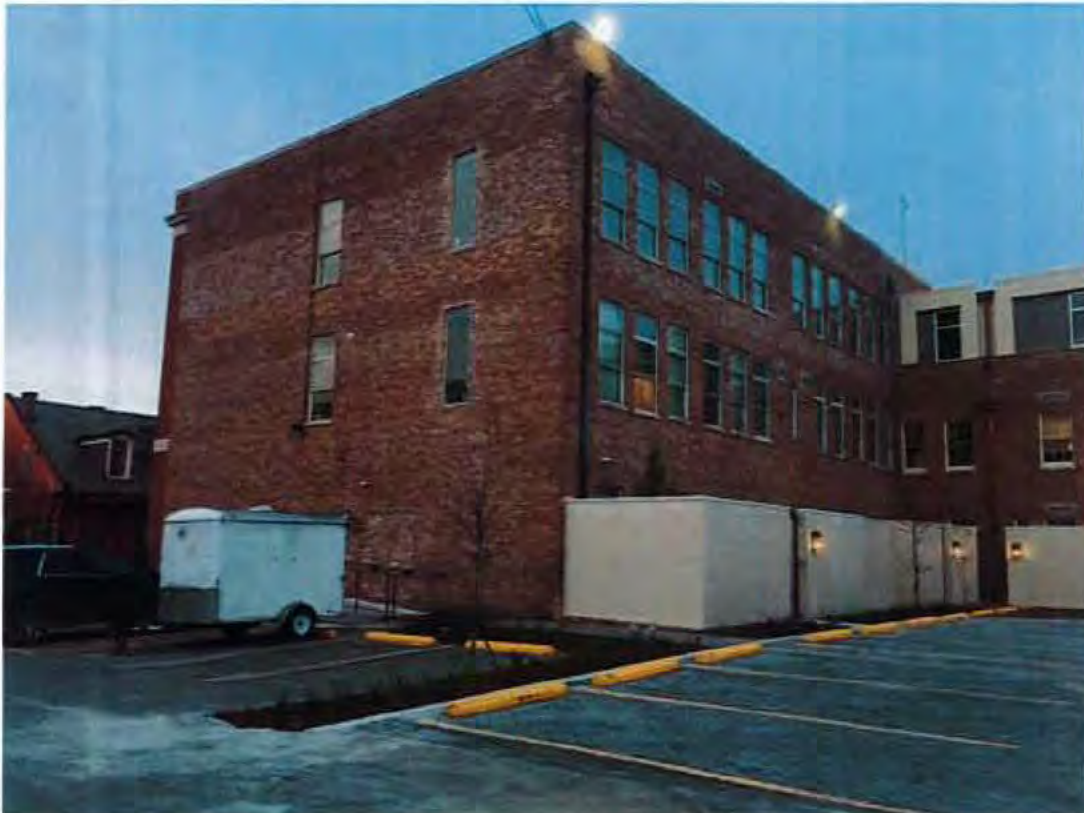
22. School, western side elevation, looking northeast
