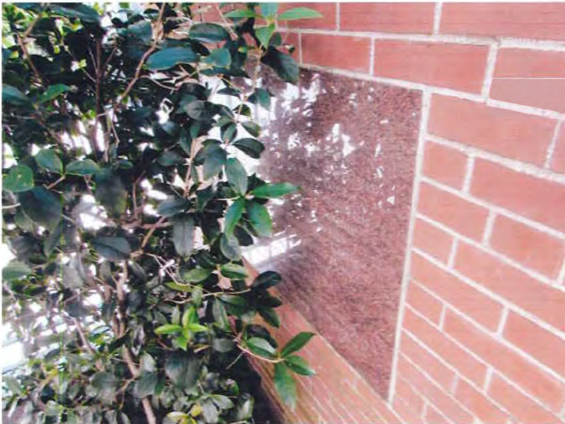
10. Cornerstone, Dauphine Street entrance, looking southeast
