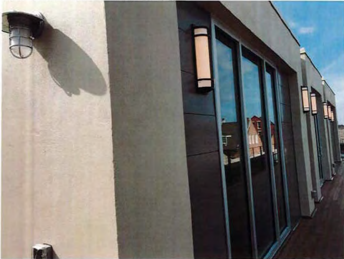
25. School, Eastern & southern elevation, looking northwest.
