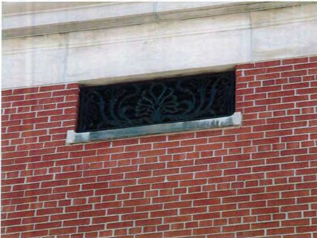
20. School, iron grille details, looking south
