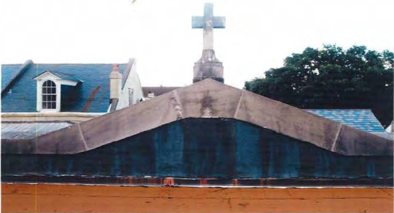
95. Convent roof, parapet, looking east
