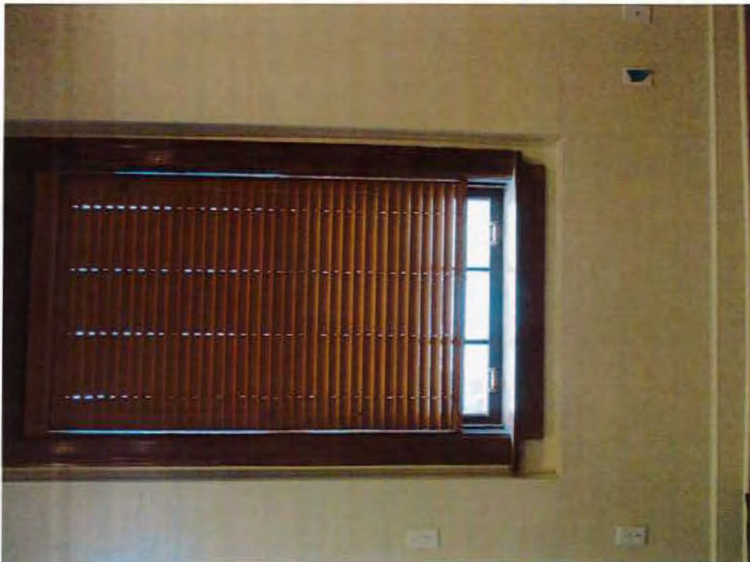
78. Convent 1 st floor, typical rear window
