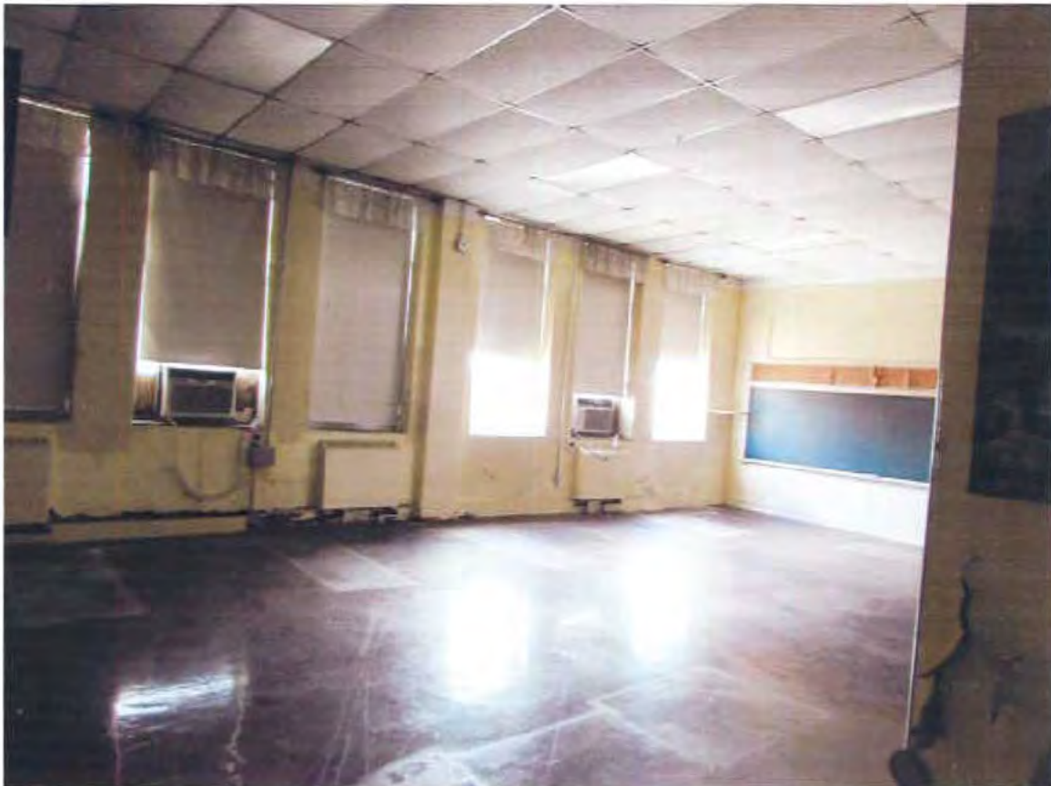
56. School, 2nd floor, front classroom 2, looking northeast
