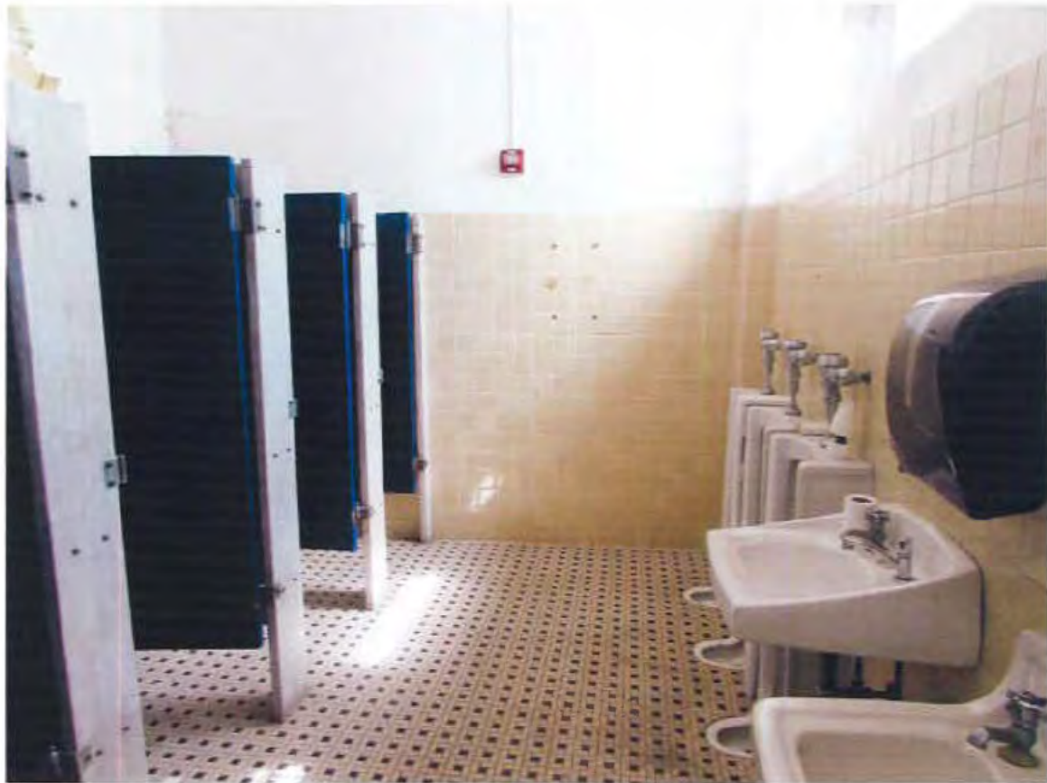
48. School, 1st floor, boys' toilet, looking southeast, looking northeast
