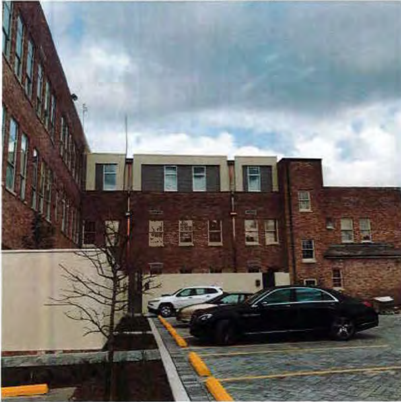
17. Convent, rear elevation, looking east
