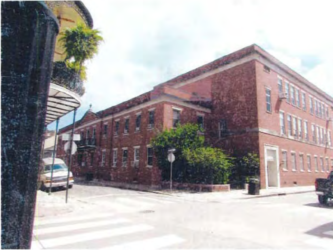
1. Dauphine & Dumaine Street Facades, looking southwest
