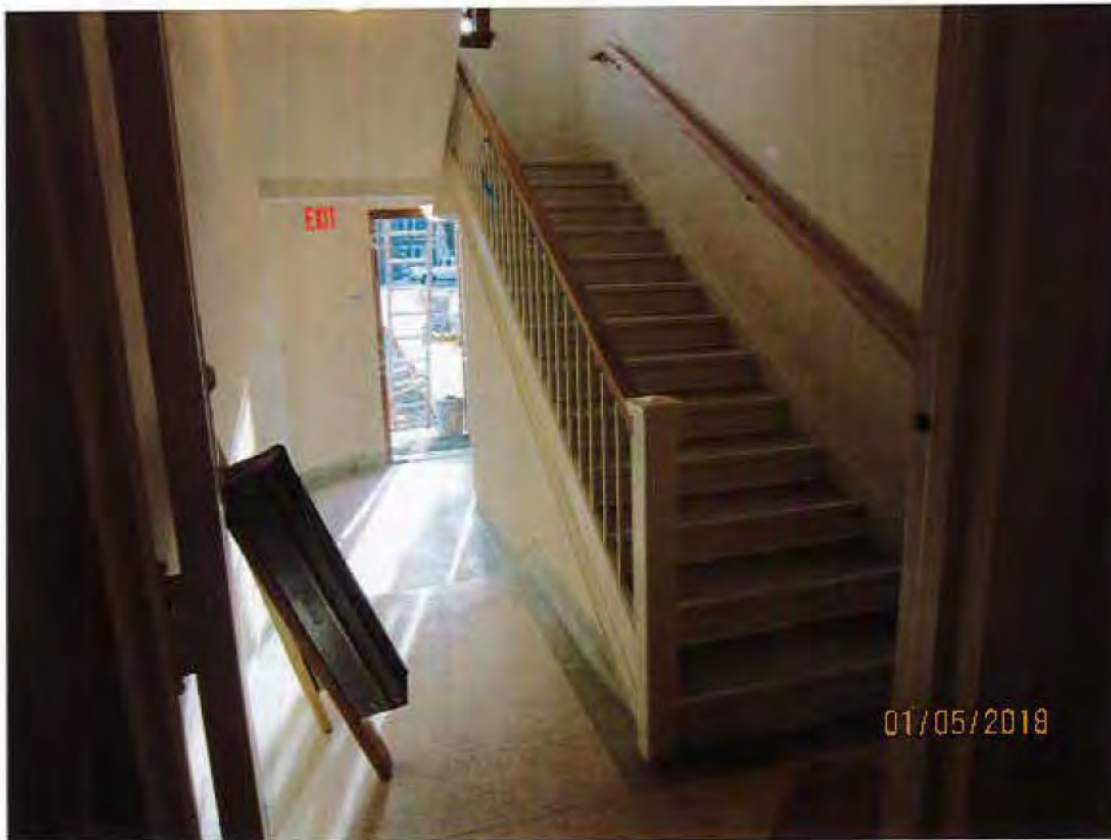
79. Convent, 1 st floor, stair, looking west
