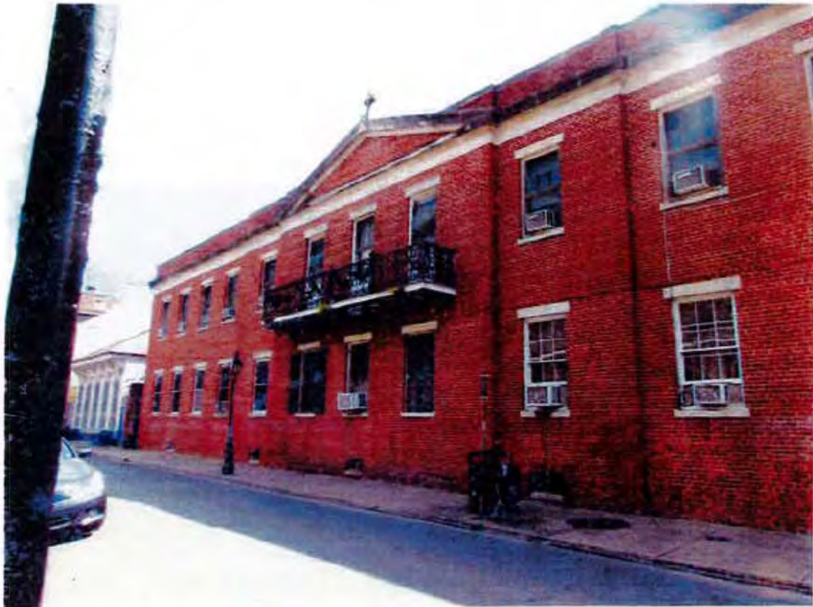
Figure 4: The North facade of the Cathedral Academy, on Dumaine Street.
