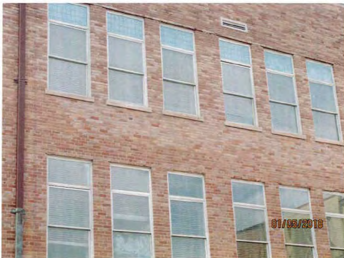
24. School, rear windows detail, looking north
