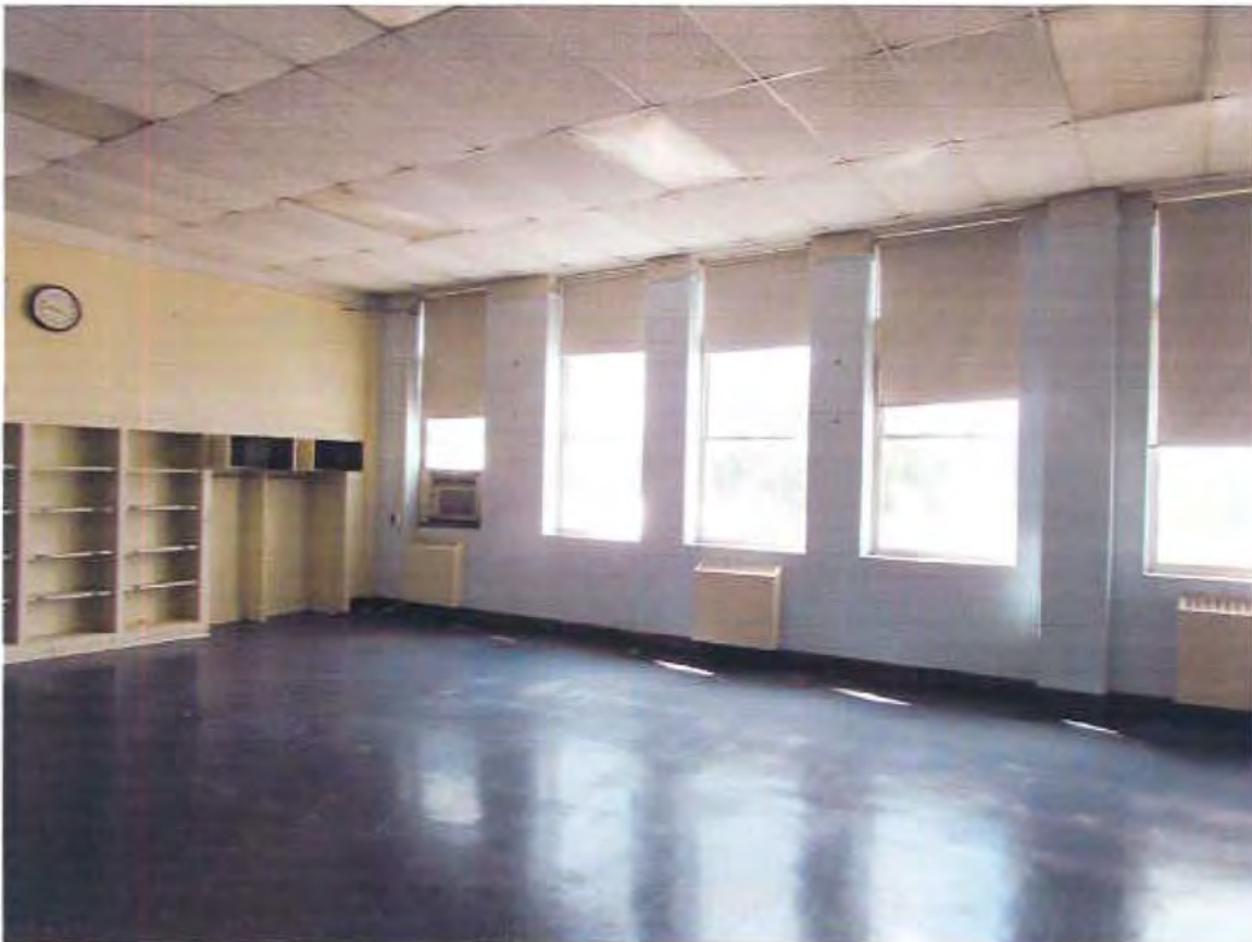
64. School, 3rd floor front classroom, looking north
