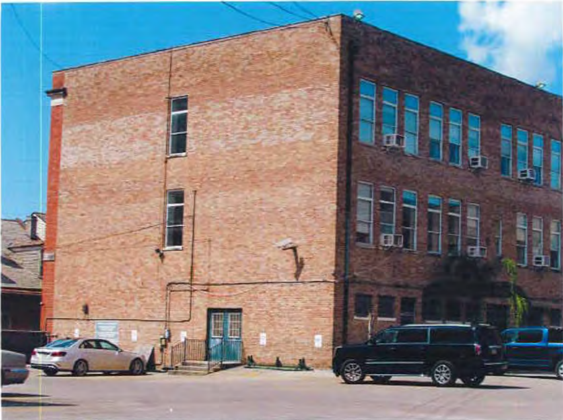
29. School, western side elevation, looking northeast
