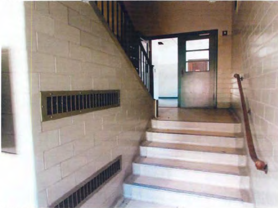
39. School 1st floor, Dauphine entry & stair 2, looking south
