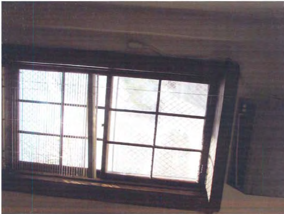
86. Convent 1st floor, typical rear window
