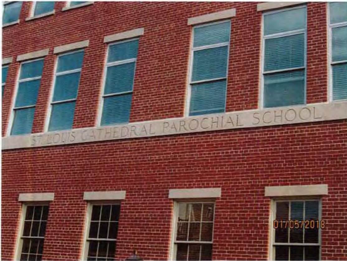
21. School. Façade detail—signage & windows
