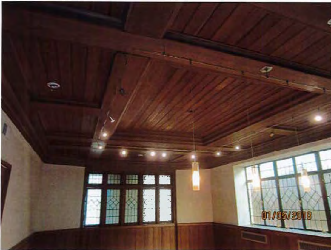
69. Chapel wood ceiling detail
