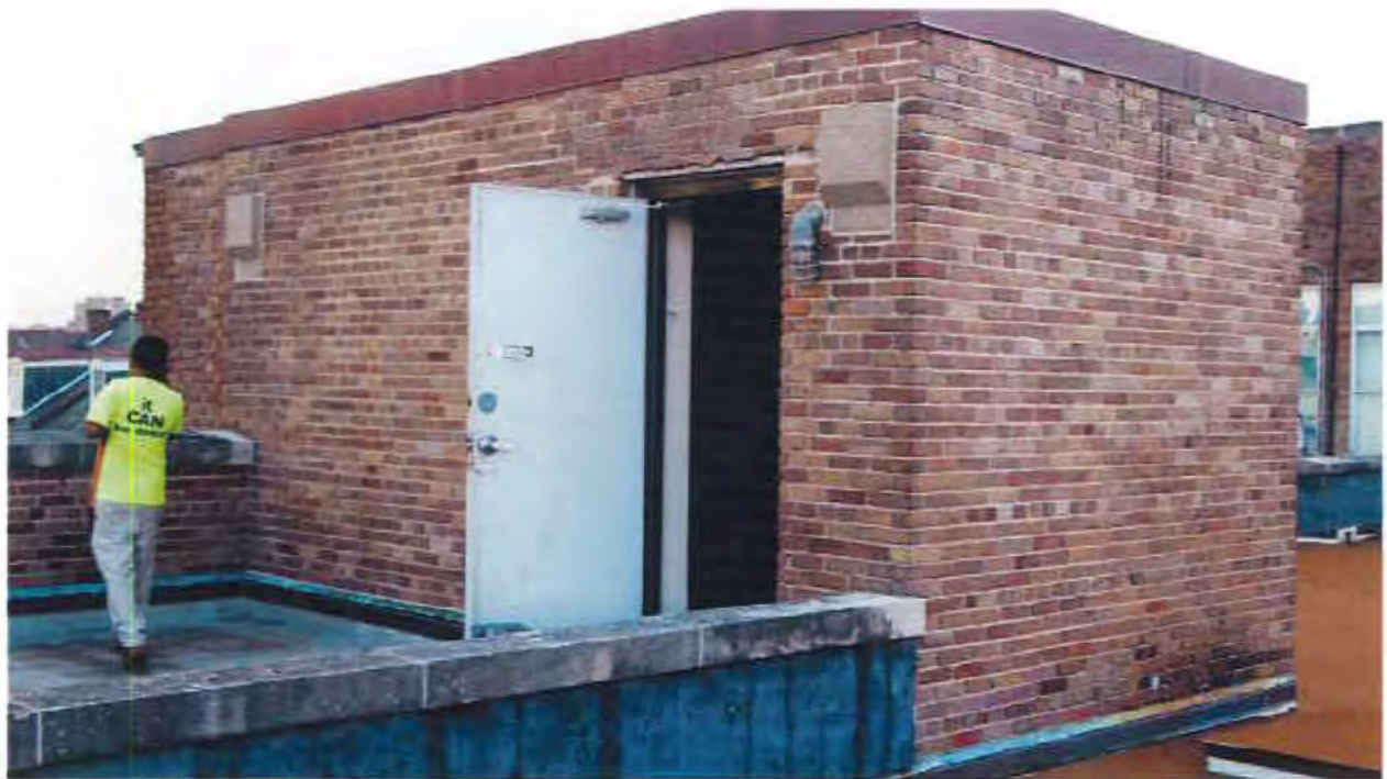
94. Convent roof, looking northwest, stair penthouse & terrace
