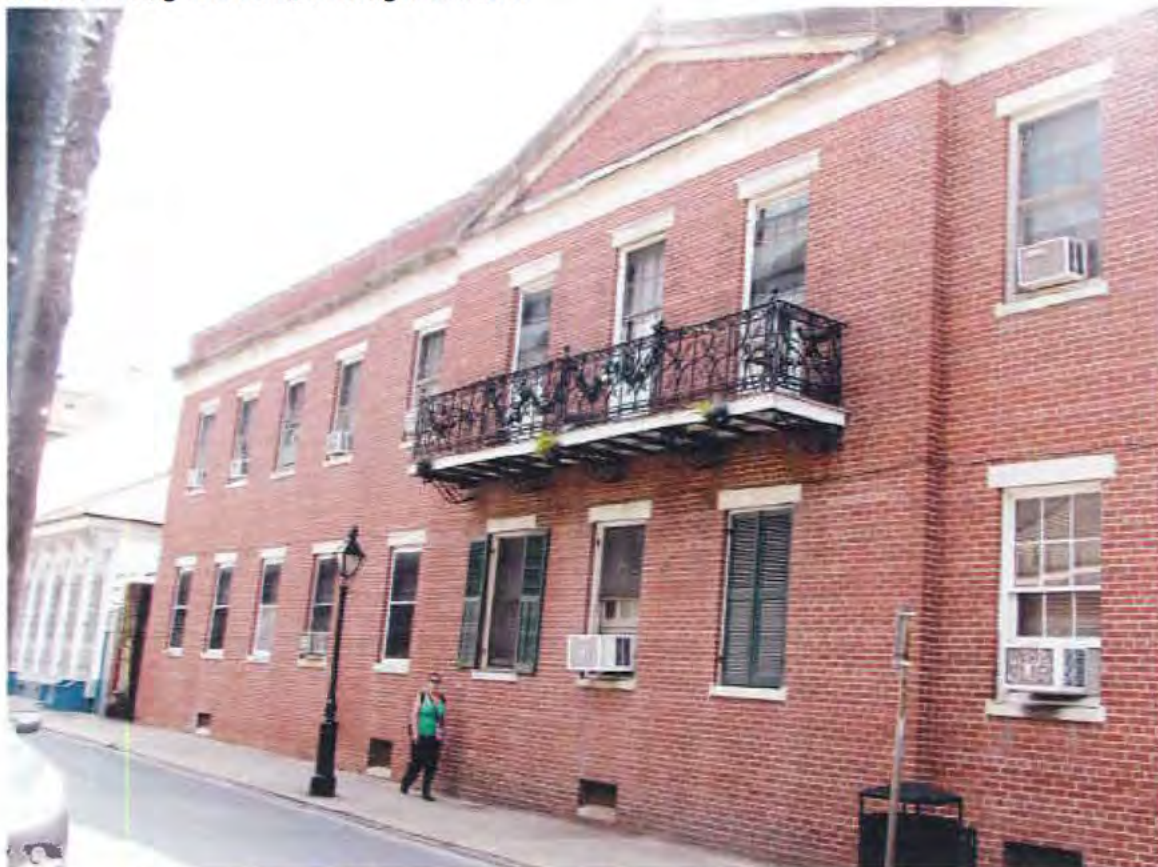
14. Convent, Dumaine Street facade, pedimented bay detail, looking southwest
