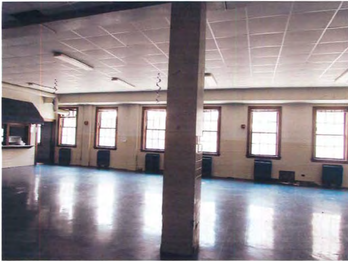
45. School, 1st floor cafeteria, looking north toward facade windows
