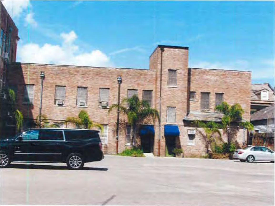
24. Convent, rear elevation, looking east
